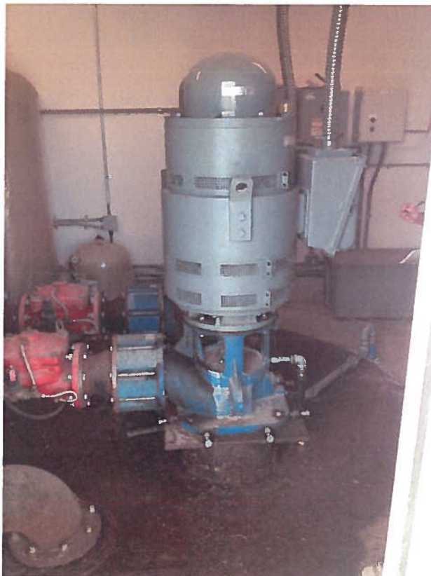
Figure 5 The pump house where water is diverted from the western pond to the irrigation system and the fire hydrants.
