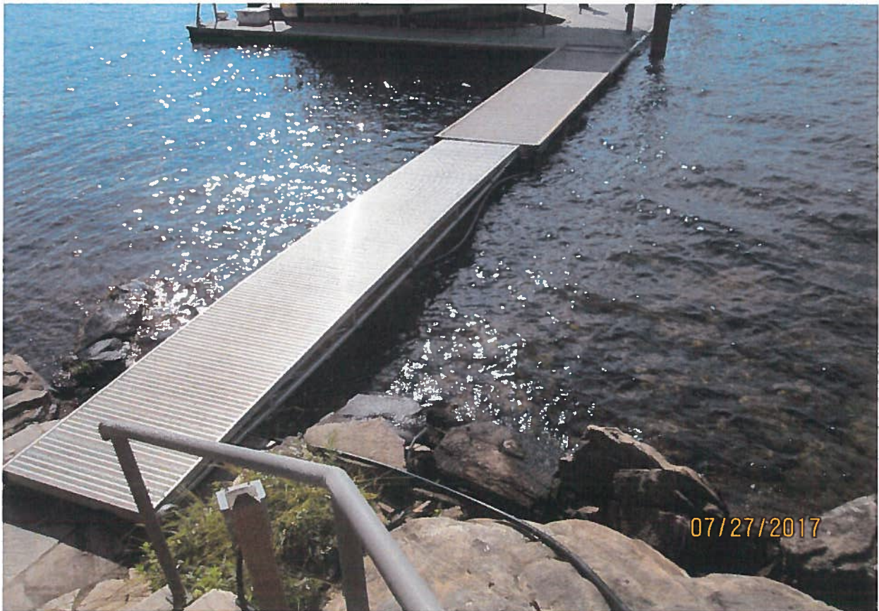
1 inch poly pipe from POD.
