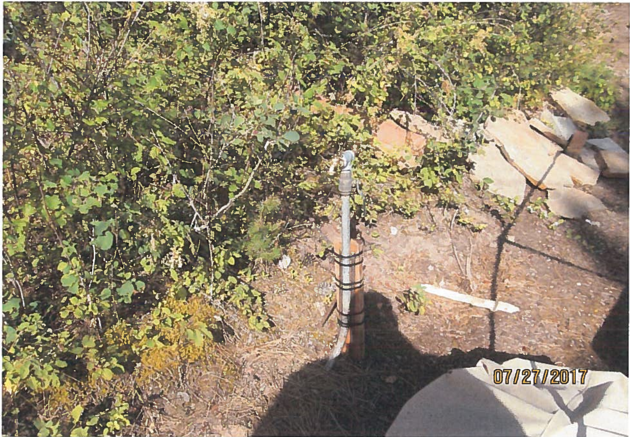
Frost free stub in on lot and place of use. 5 gallon bucket test performed in 32 seconds or 9gpm or 0.02 cfs.
