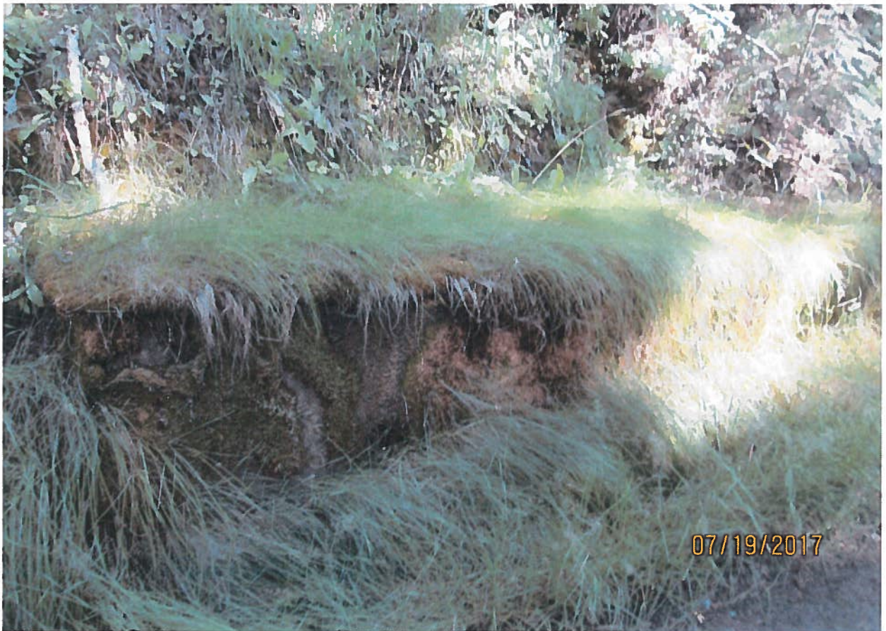
POD, very old spring box with grass growing all over.
