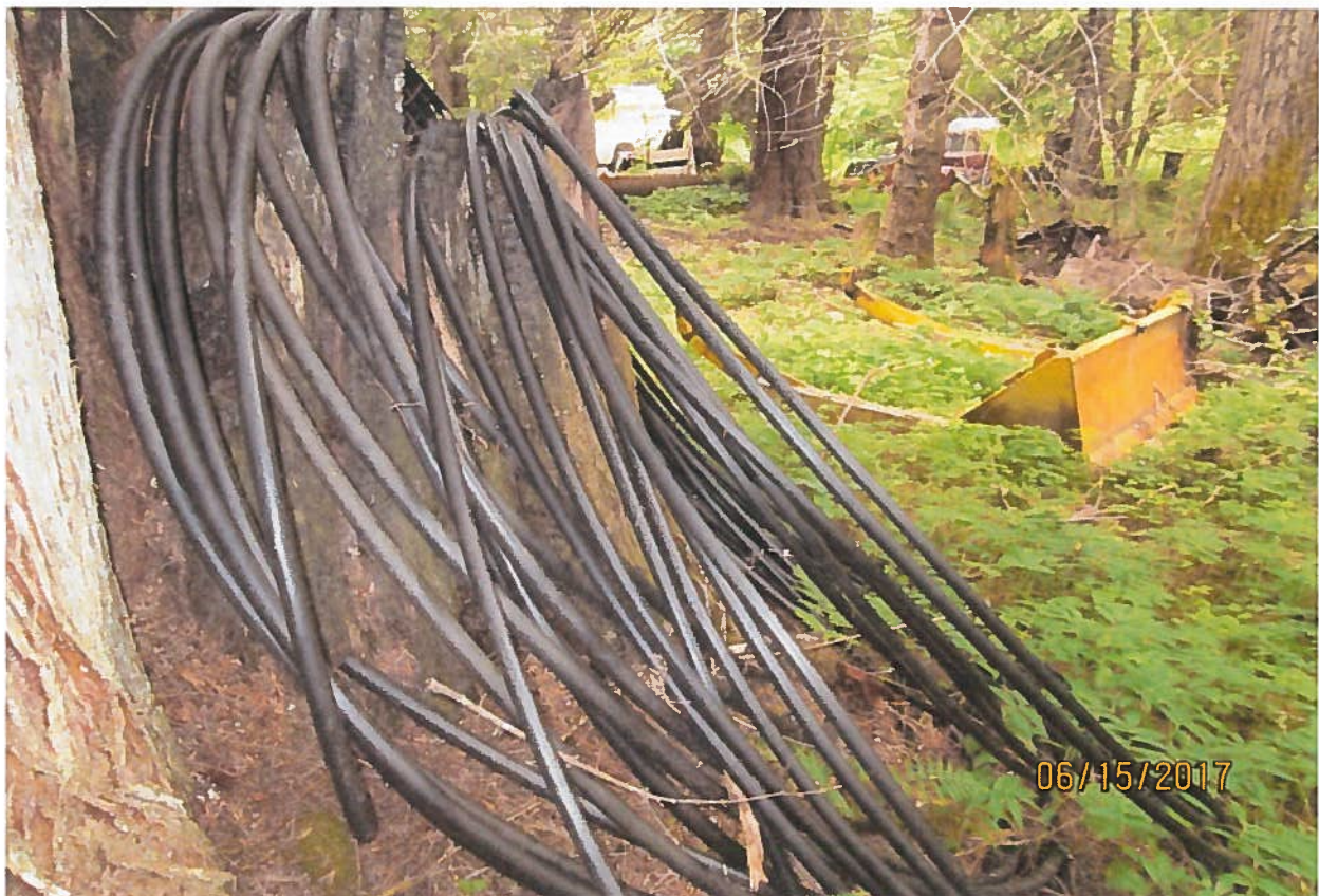
Applicant would lay down pvc pipe if bulldozer could not get close to new plantings.
