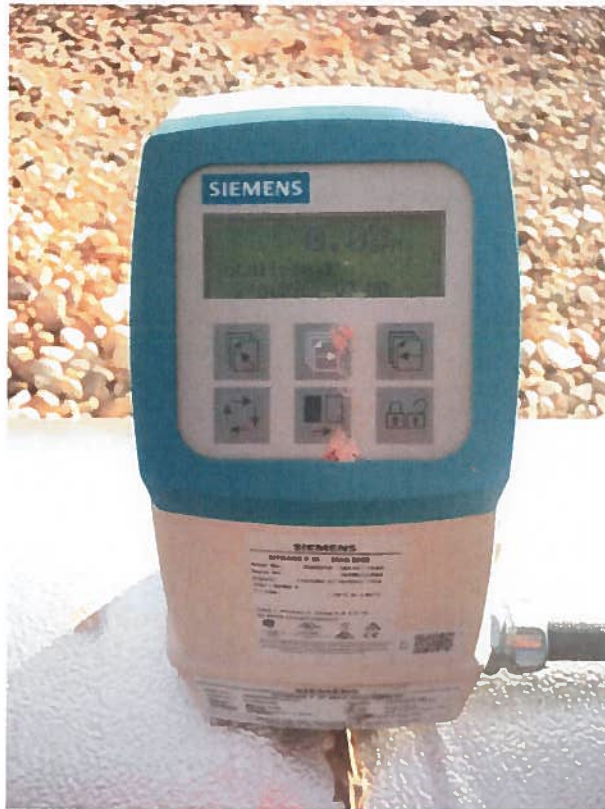
Irrigation Well No. 3 Totalizer (11/17/2017)
