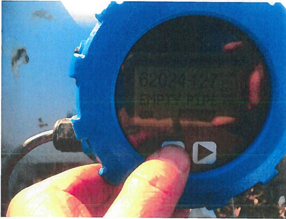
Irrigation Well No. 1 Totalizer (11/17/2017)
