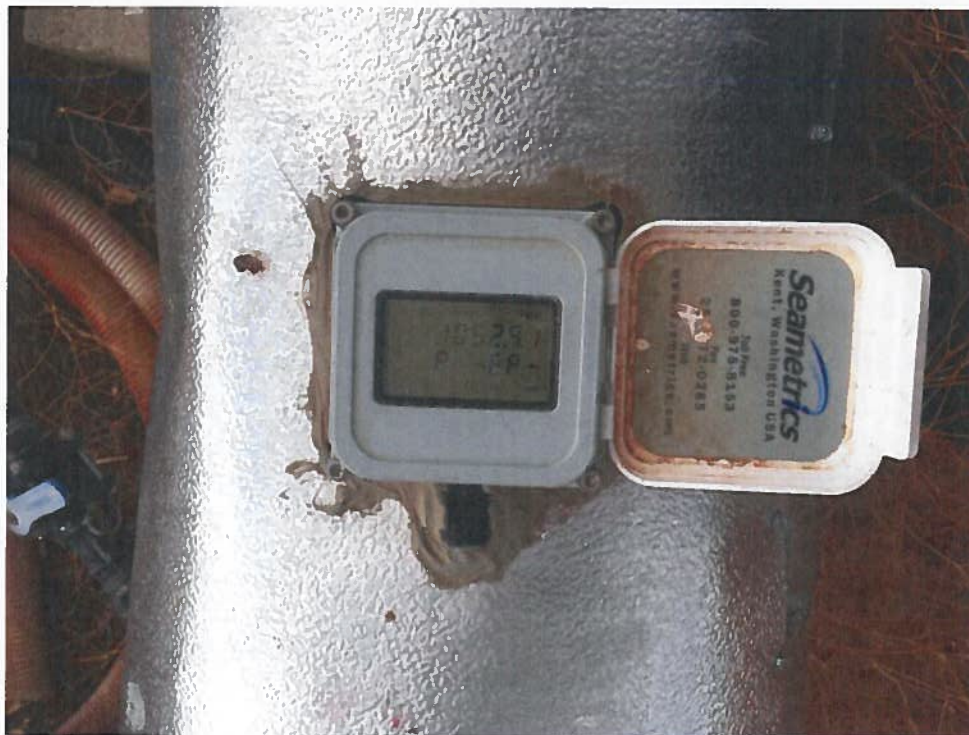
Irrigation Well No. 2 Totalizer (11/17/2017)
