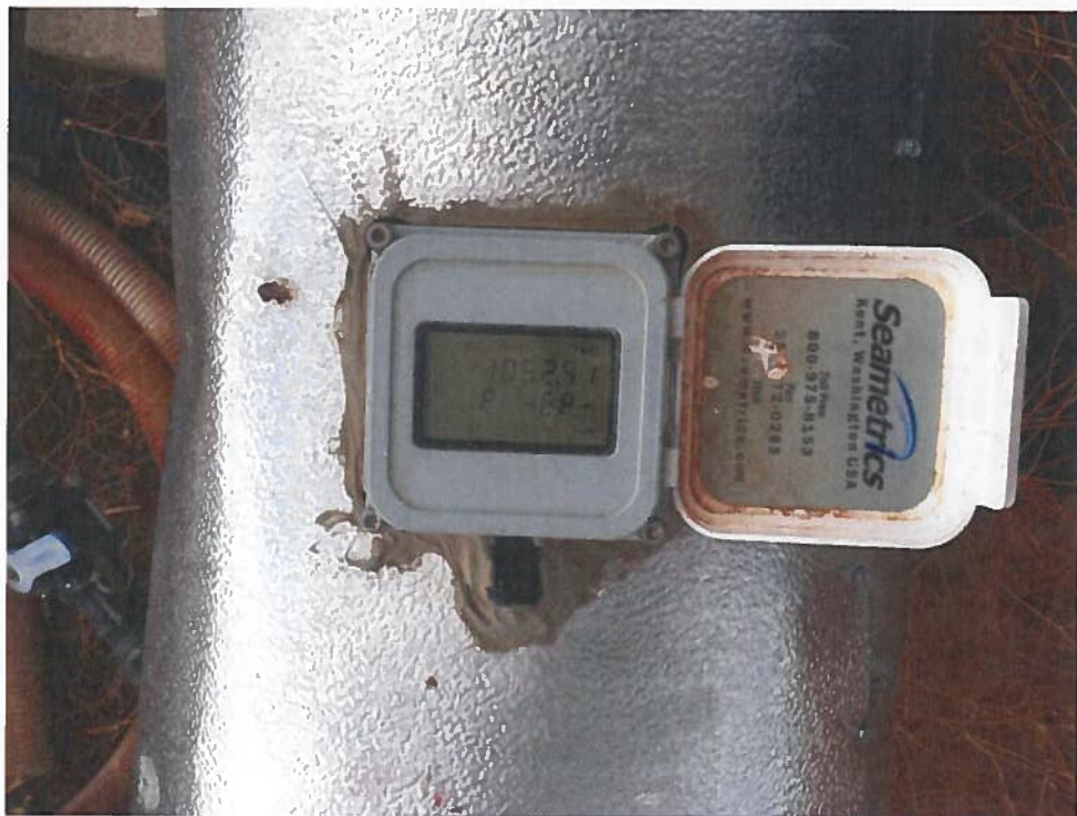
Irrigation Well No. 2 Totalizer (11/17/2017)
