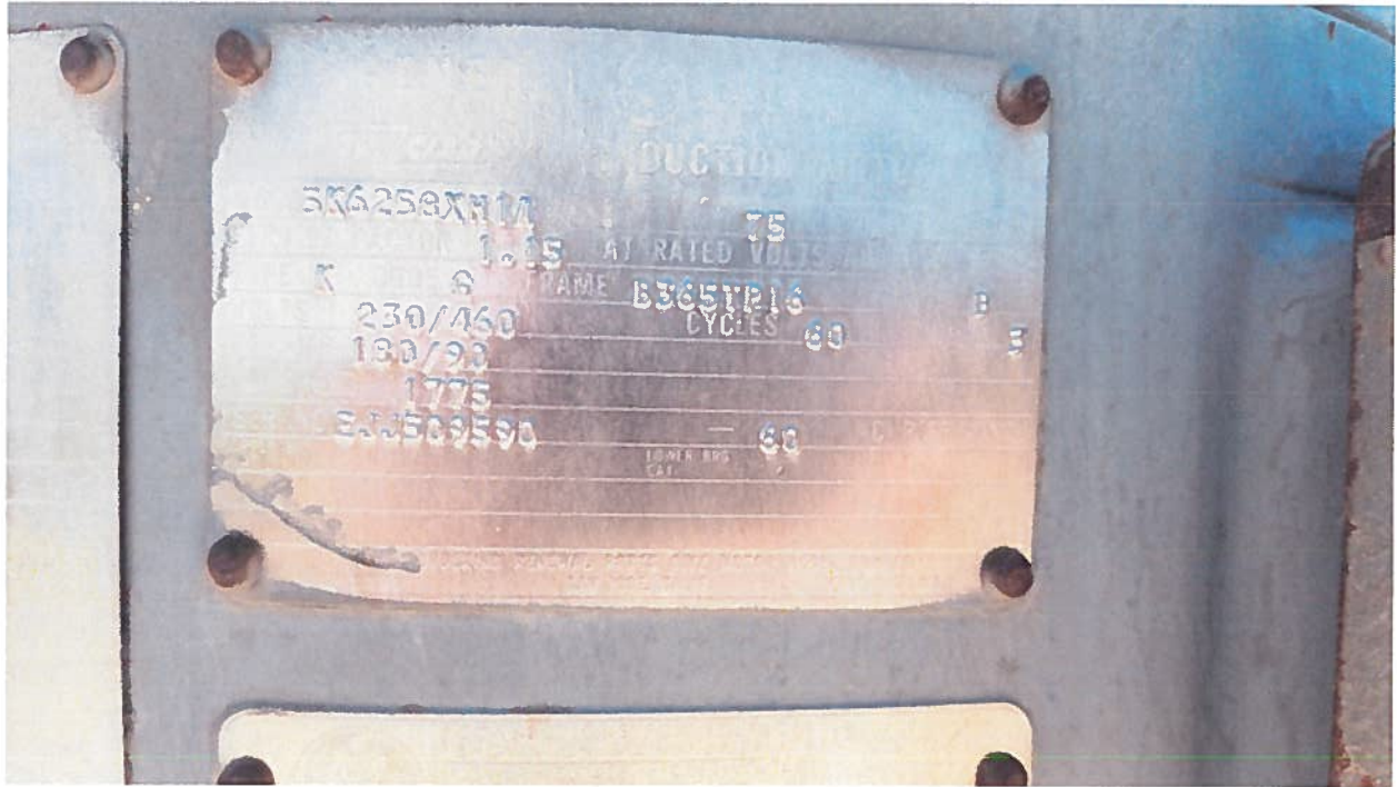
Picture 5. The motor plated mounted on the Lower Well.
