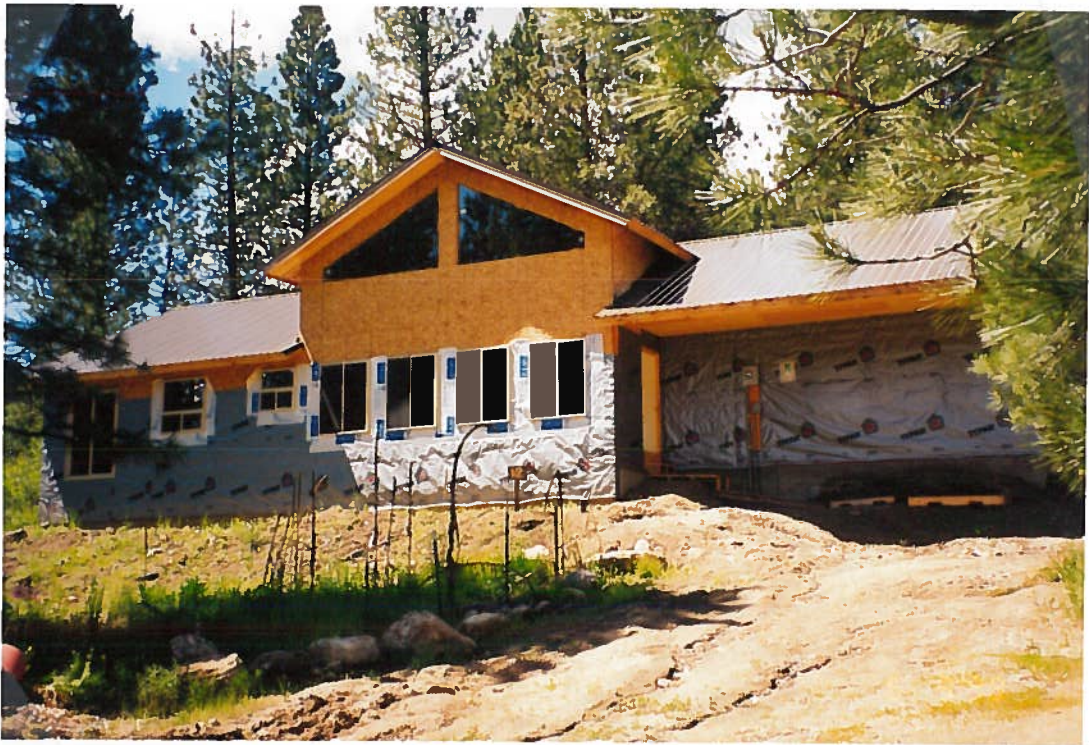
Picture 1. House under construction on Lot 2 Livingston Estates #1. This is part of the place of use for the Heating and Domestic use.
