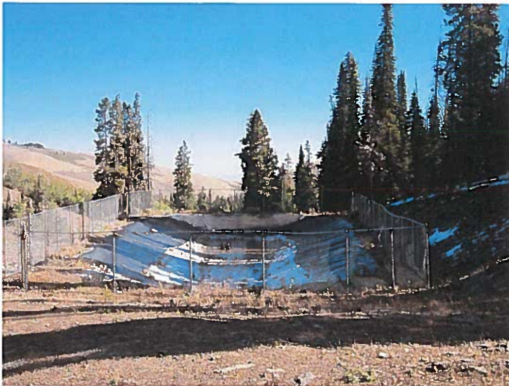
Figure 6: Storage pond below storage tank. Note that the pond is not located on a channel.
