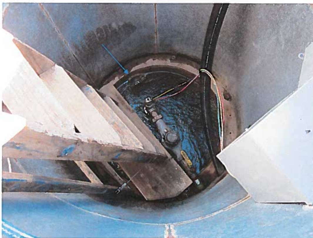
Figure 9: Looking into diversion at Bennett Spring (notice bypass just above meter).
