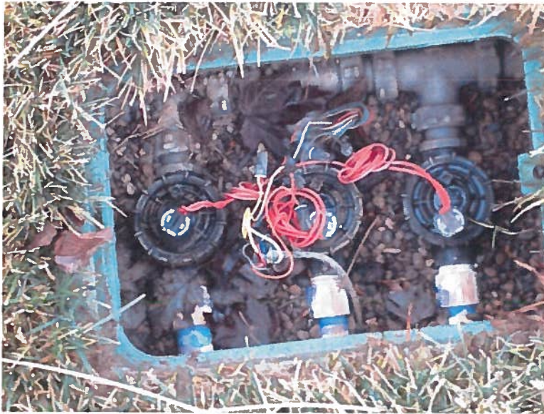
Figure 3 Irrigation valves controlled by the RainBird timer
