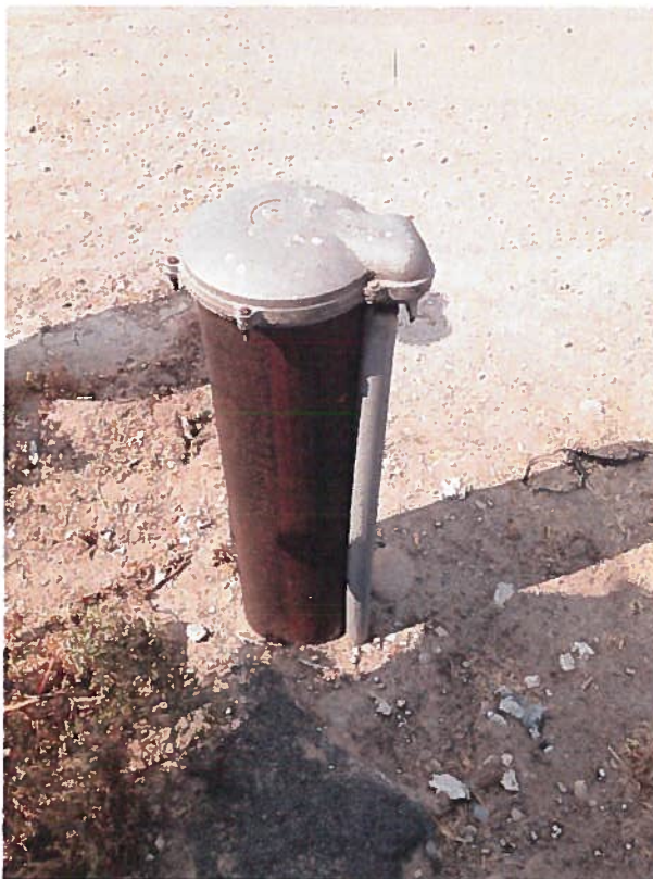
Figure 2 The southern POD located at the southeast corner of the property along County Line Rd.
