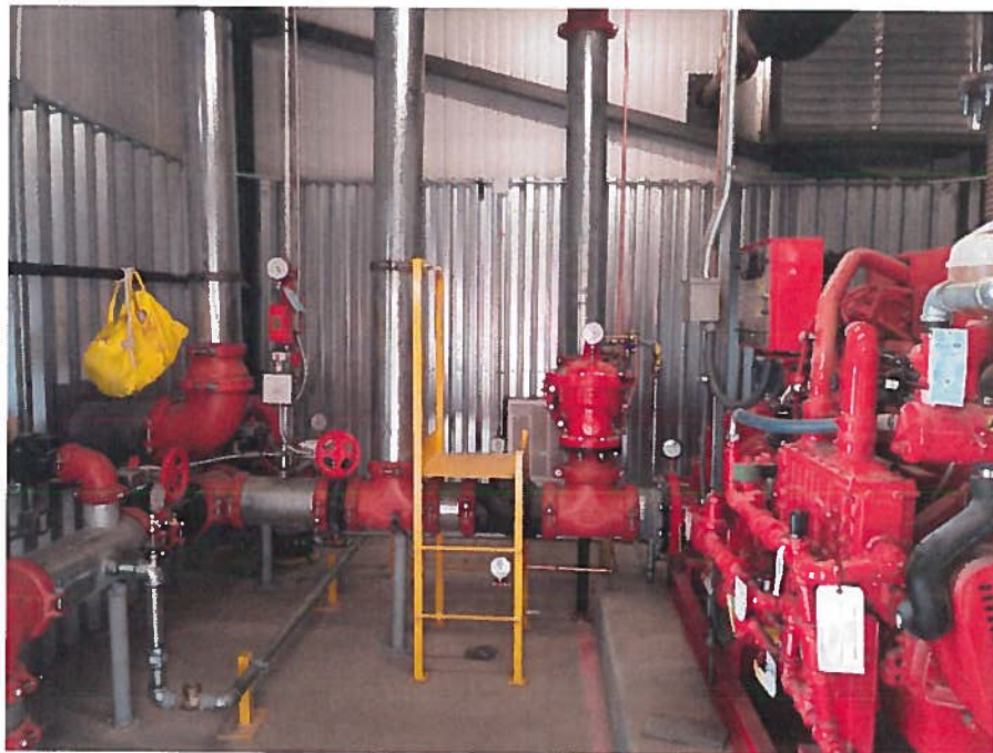
Figure 2 Inside the pump house
