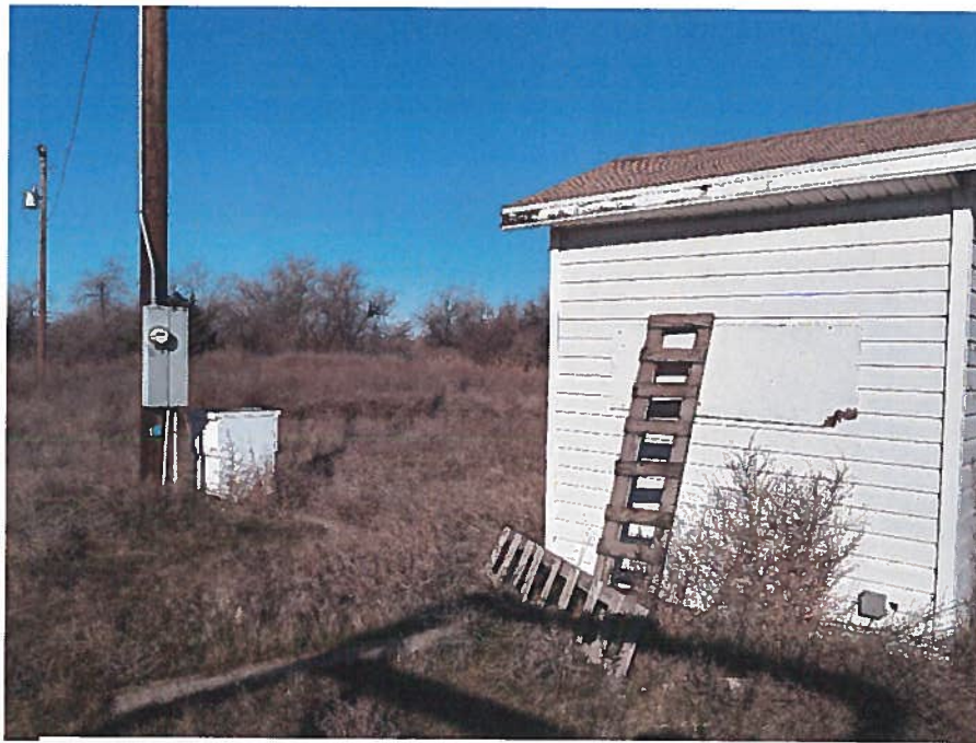
Figure 4 This shed may have been for changing or for storage. There also appears to be power at the site though nothing is operating at this time.
