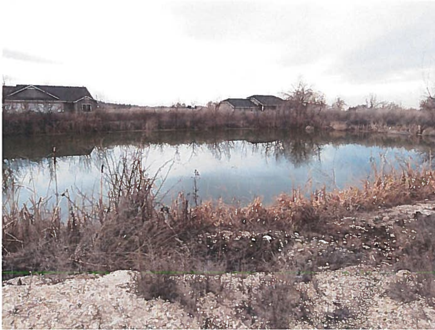
Figure 1 Fire protection storage pond in the SENE QQ. The pond is around 0.41 acres at the surface with a maximum depth of 17 ft.
