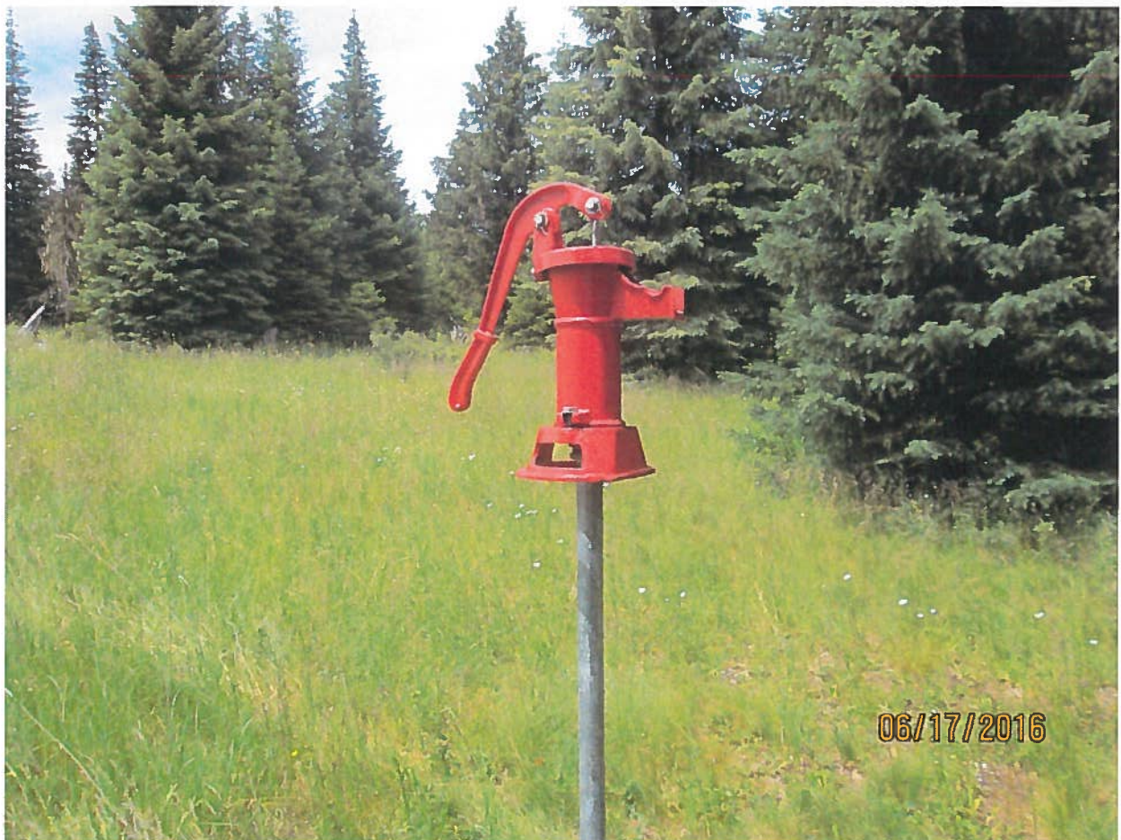
Spring source that applicant had built spring box down below the surface and put a pump hydrant on top and ran a water line to house.
