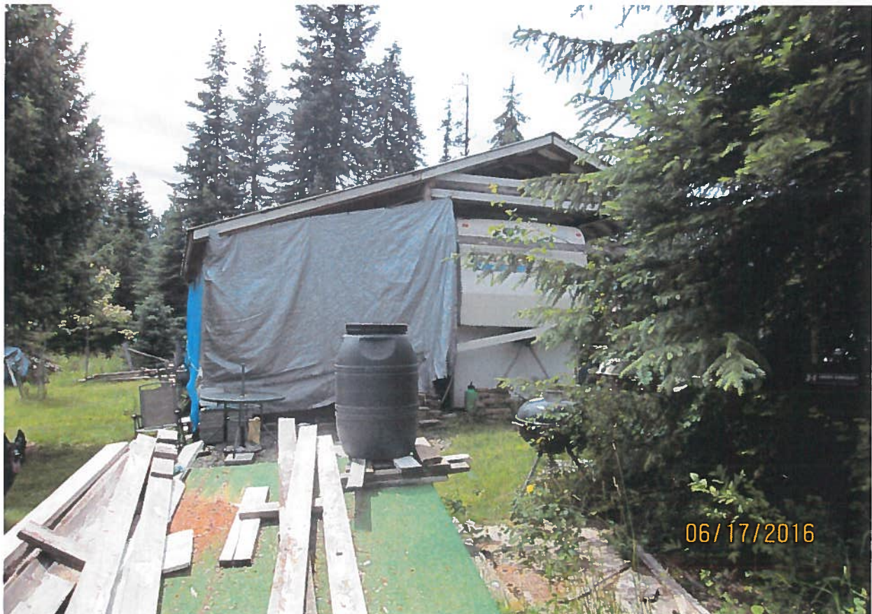
Applicant's home while he built the permanent structure.
