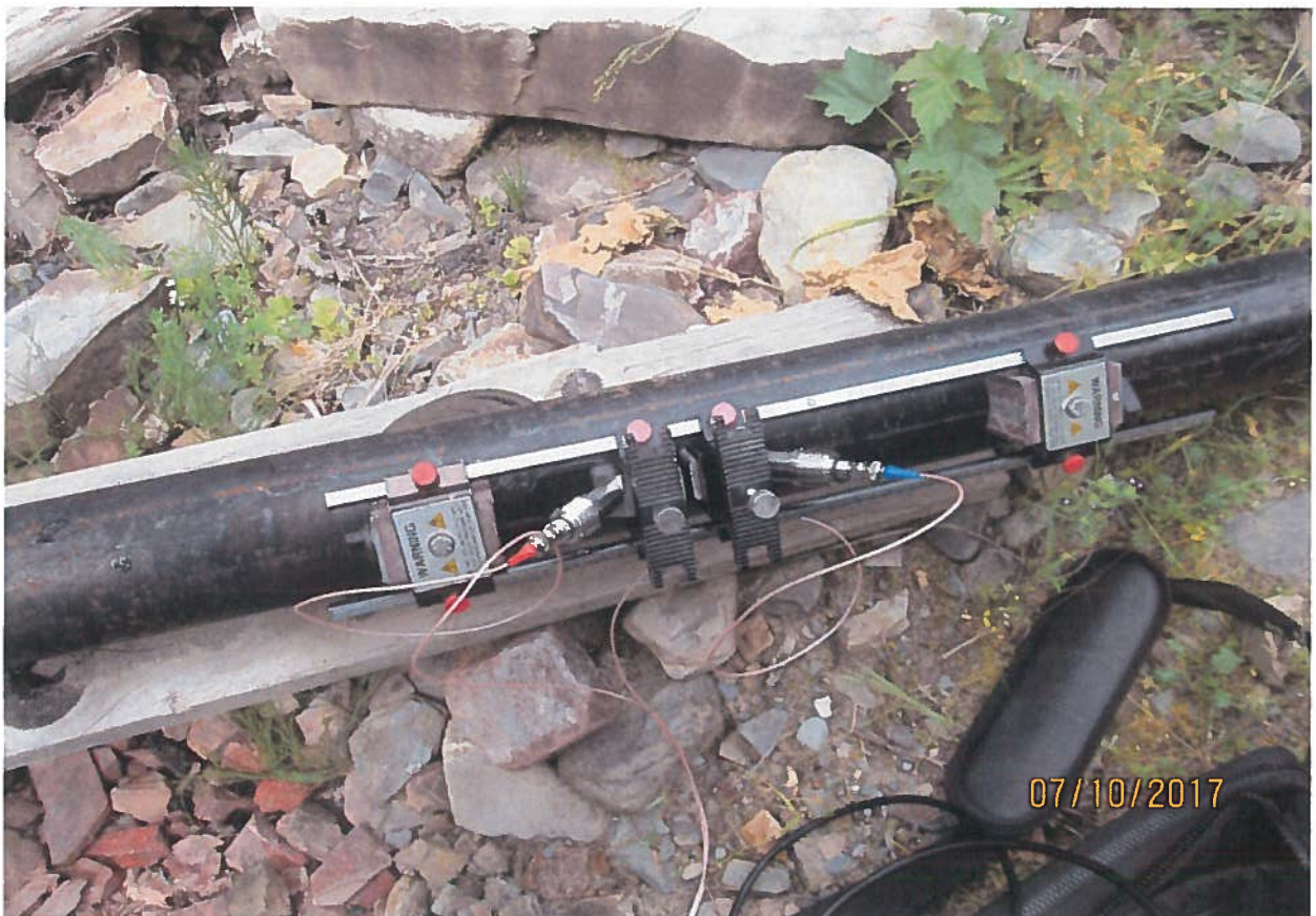
Flow measurement performed using GE Panametric Meter.
