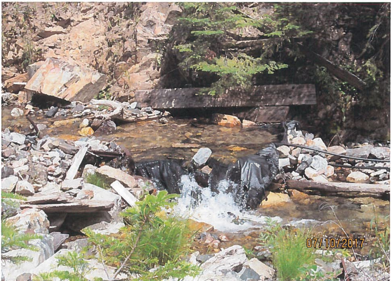
Upper POD for gravity fed system. Applicant had installed 1,300 feet of piping.
