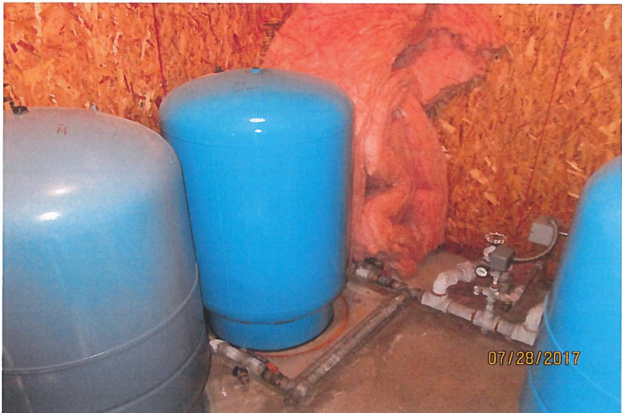
From the storage tank, water would be pumped into pressure tanks for distribution to homes.
