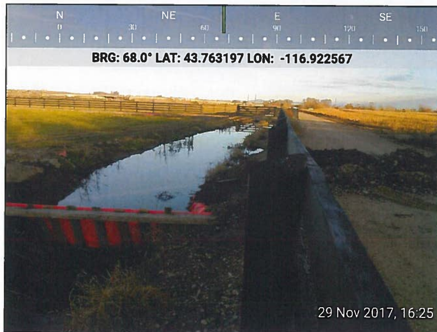
Figure 8: Flow checked to discharge into Russian Olive area. Pump station in far background.
