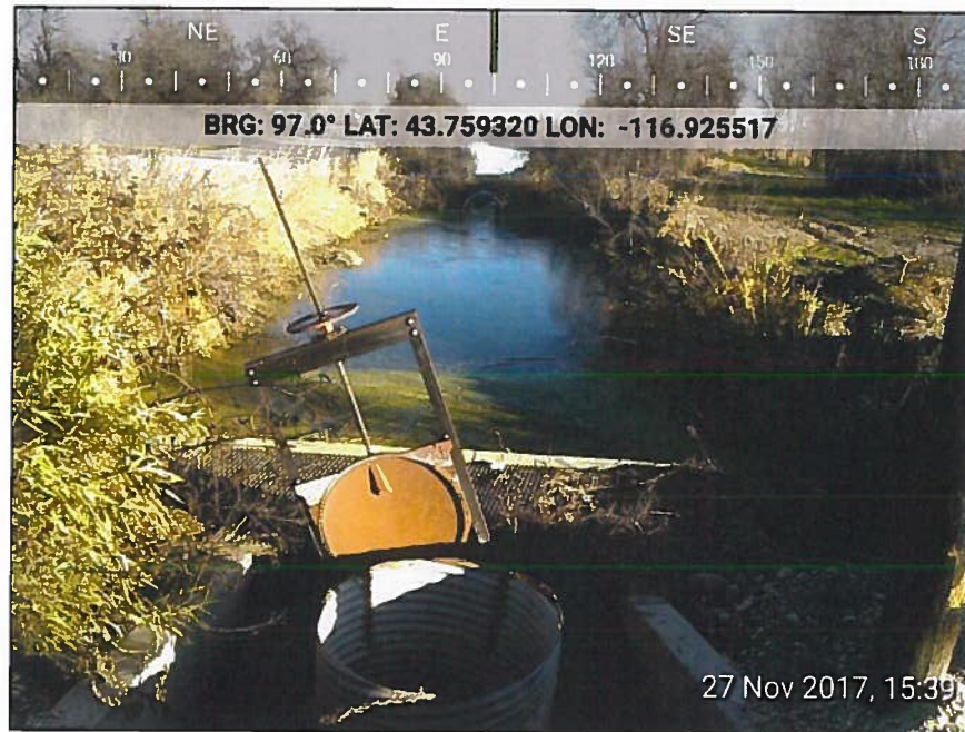
Figure 5: Lower end of Boise River source water collection ditch and entrance to pipeline under Parma Ditch.
