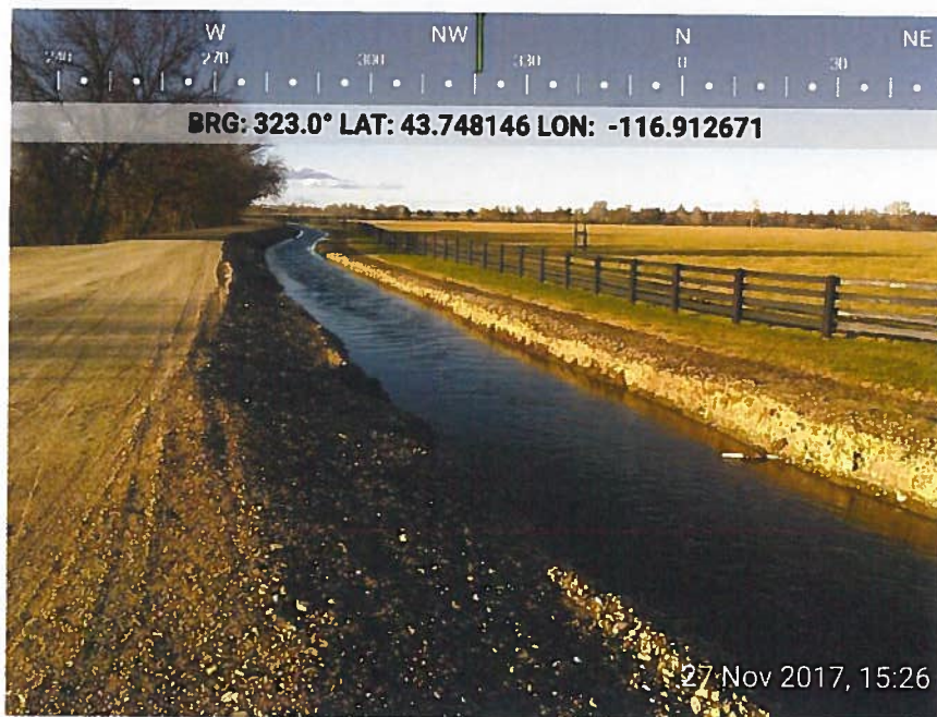
Figure 4: Same location as above figure facing northwest .
