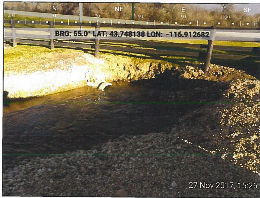
Figure 3: Andrews Ditch flow entering Tree Top Ranches property on west side of Hwy 95.
