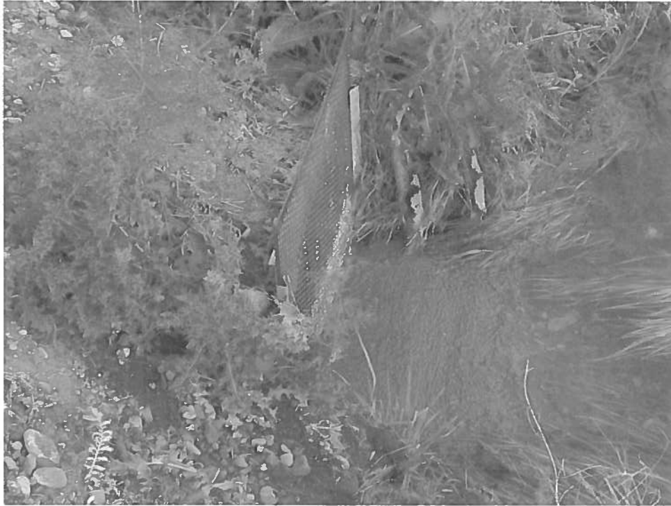
West Pond - 24" CMP Outlet - Ungated
