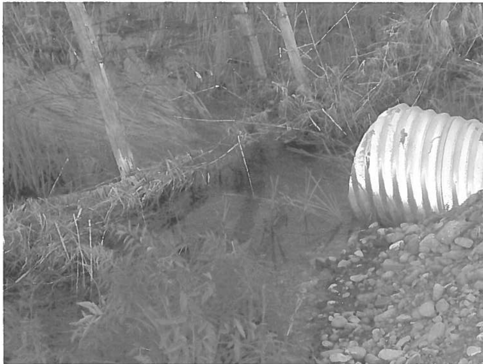
West Pond - 24" CMP Outlet - Note flowing water.
