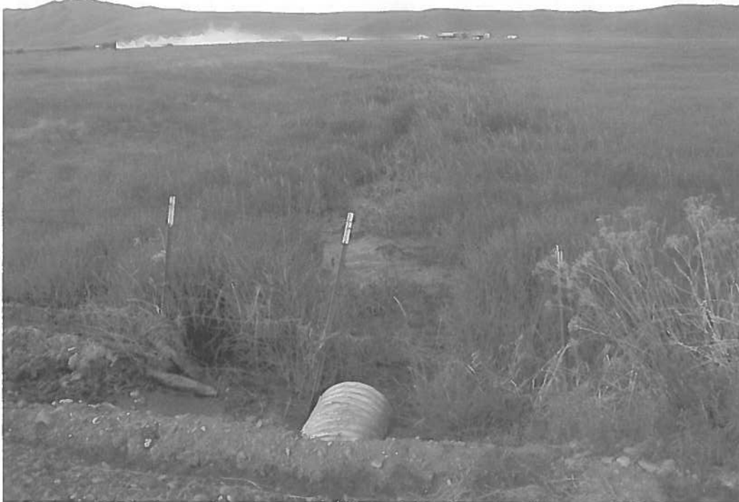
East Pond - 18" CMP Outlet - Looking downstream at swale
