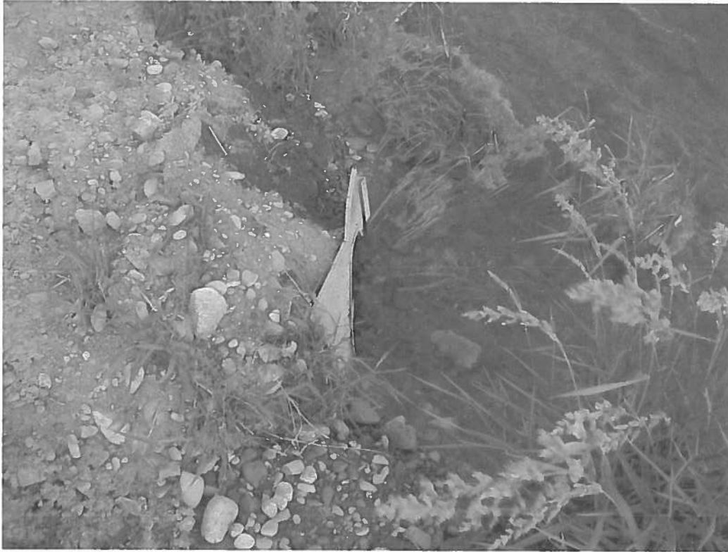
East Pond - 18" CMP Outlet - Ungated
