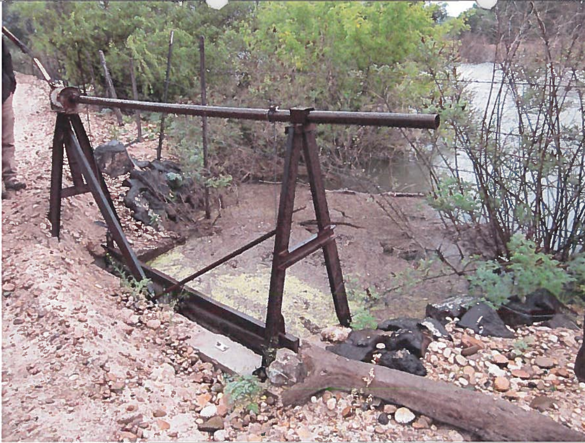
Point of Diversion from the Boise River.
