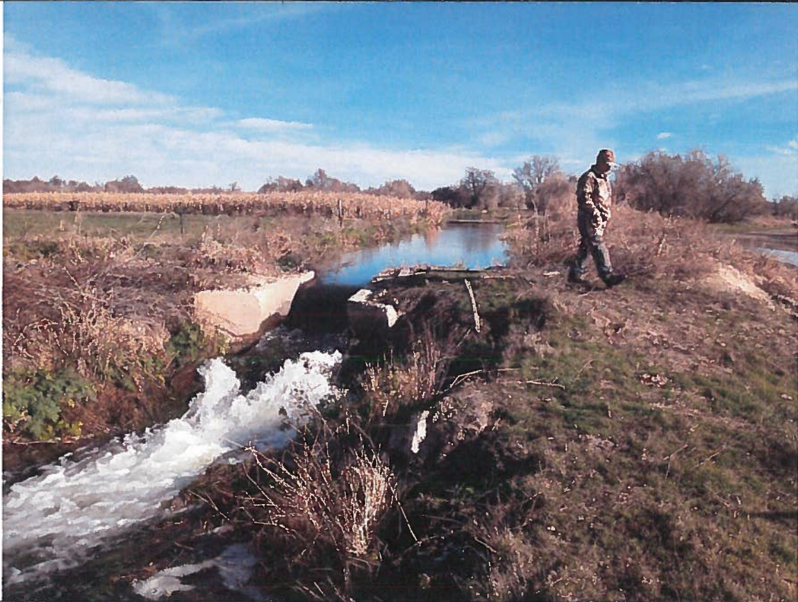
Calculated as a compressed rectangular weir producing a discharge of 9.15 cfs. 4' width X 0.8' depth.
