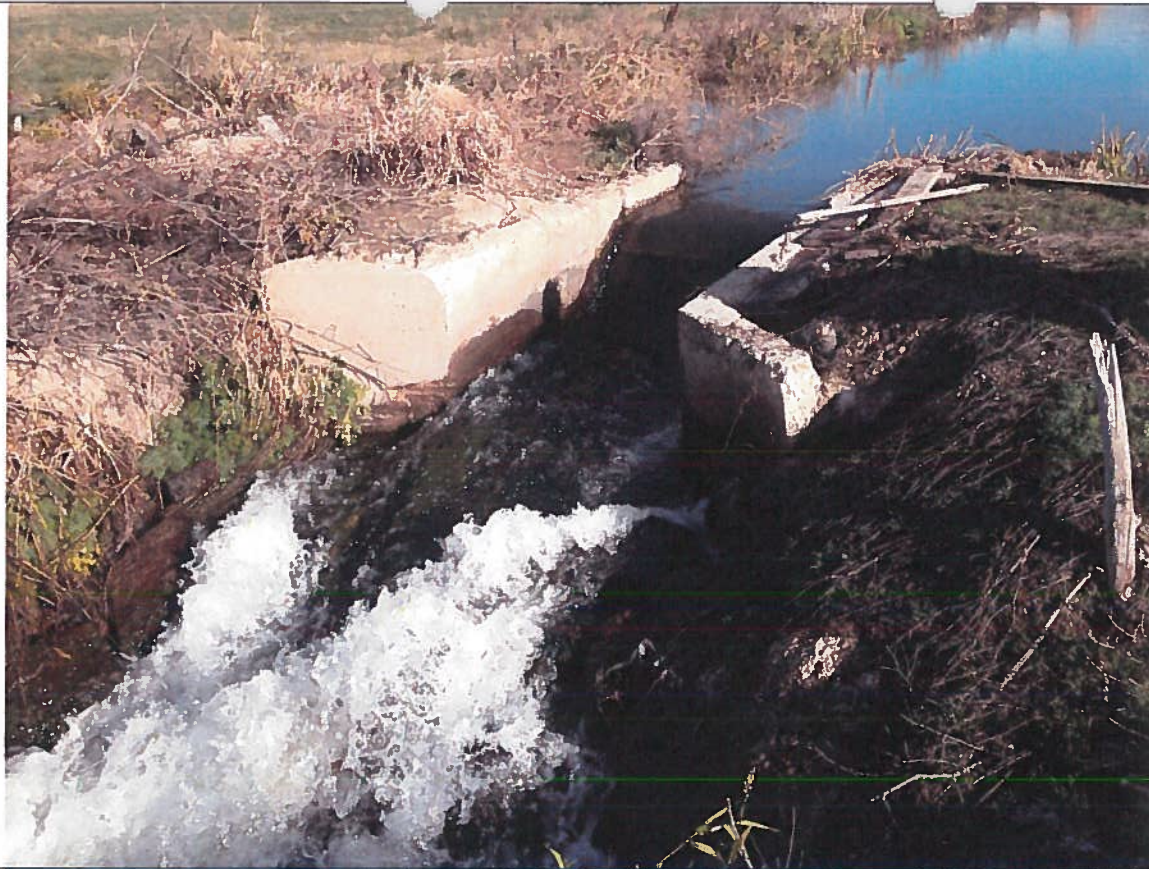
Andrew Ditch End Weir located at ~ 43°44'44.94" N 116°53'37.08" W.
