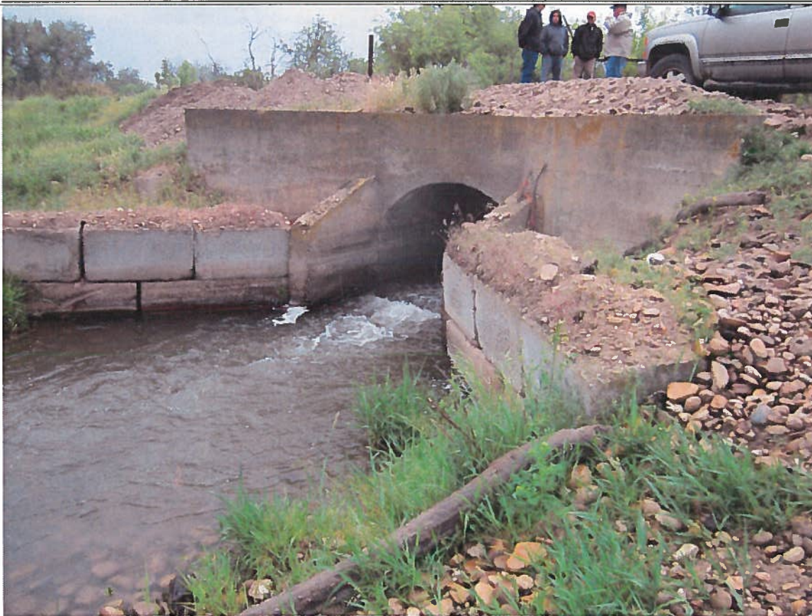
6' concrete arch diverting water into Andrew Ditch.
