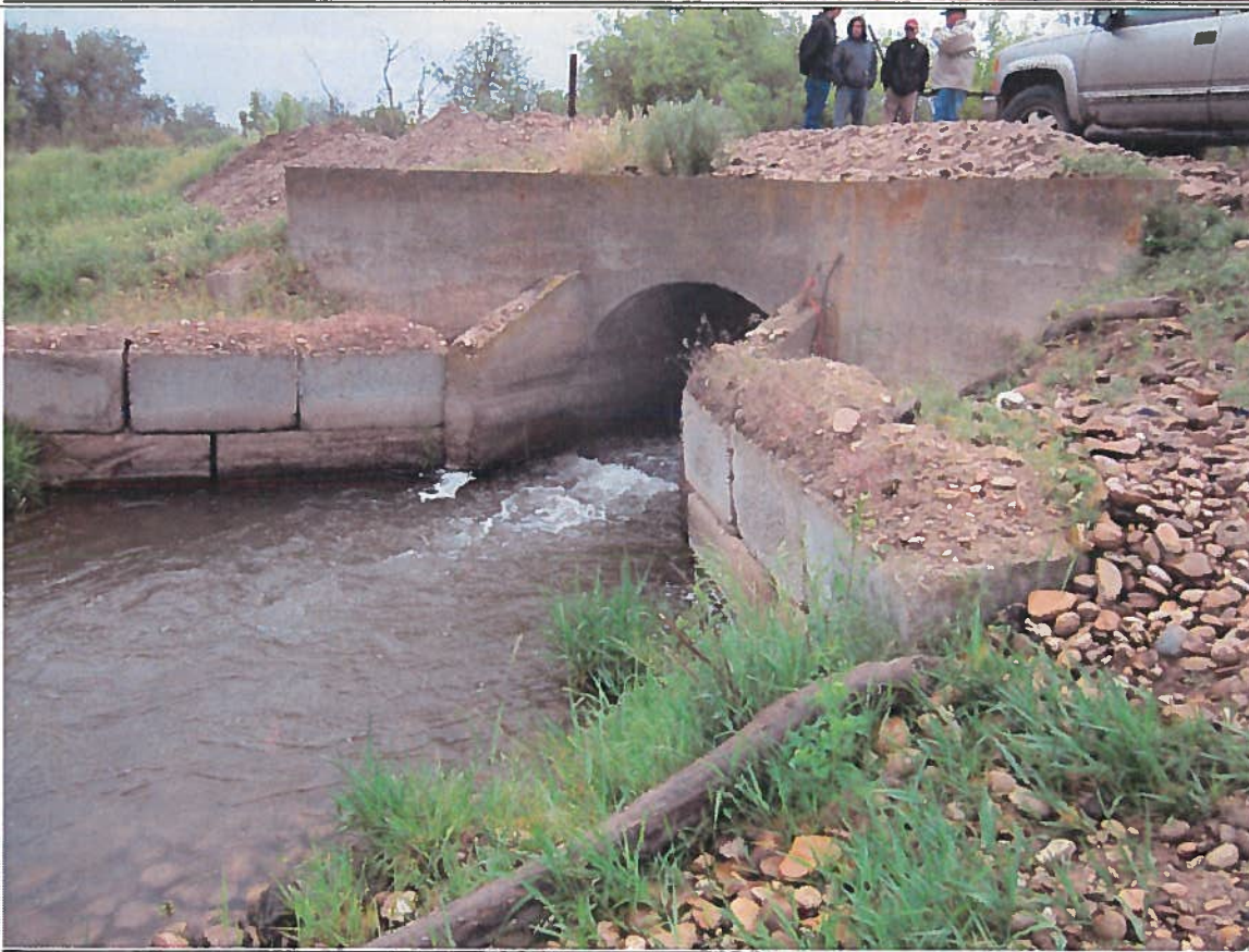
6' concrete arch diverting water into Andrew Ditch.
