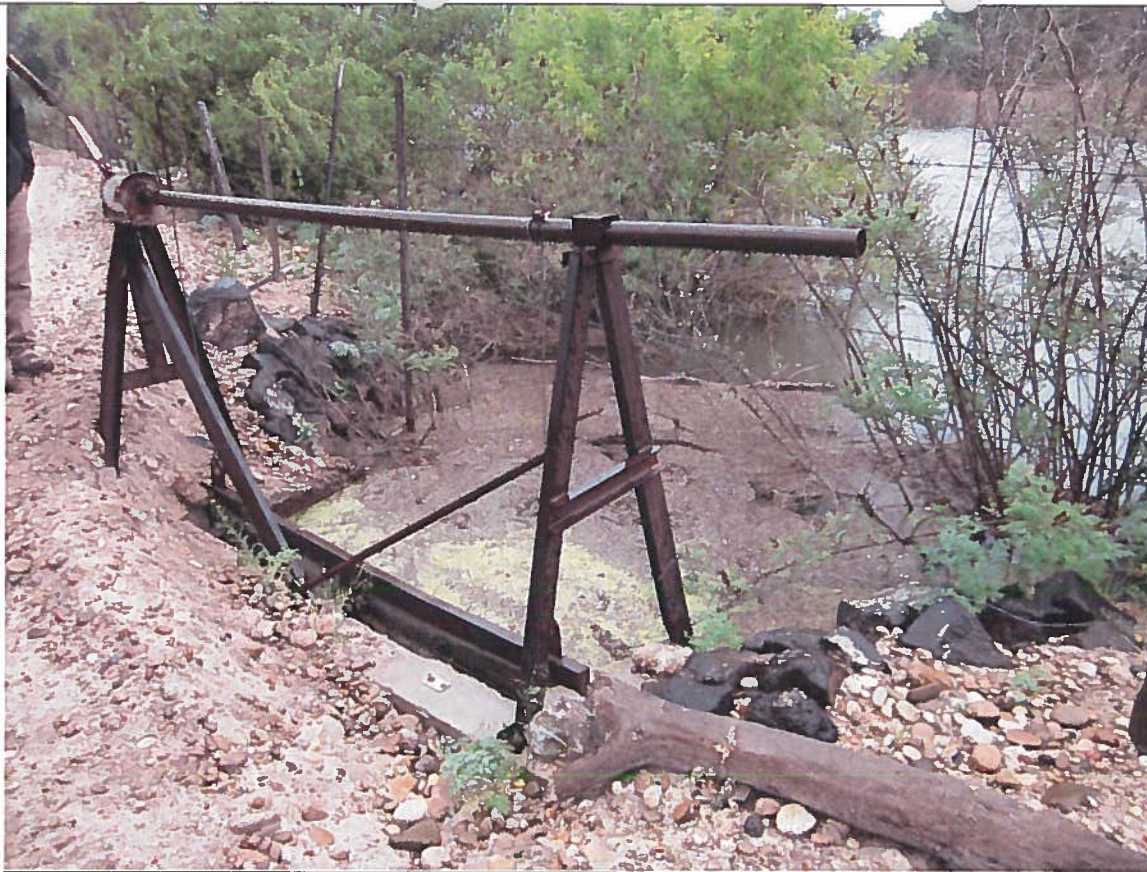
Point of Diversion from the Boise River.
