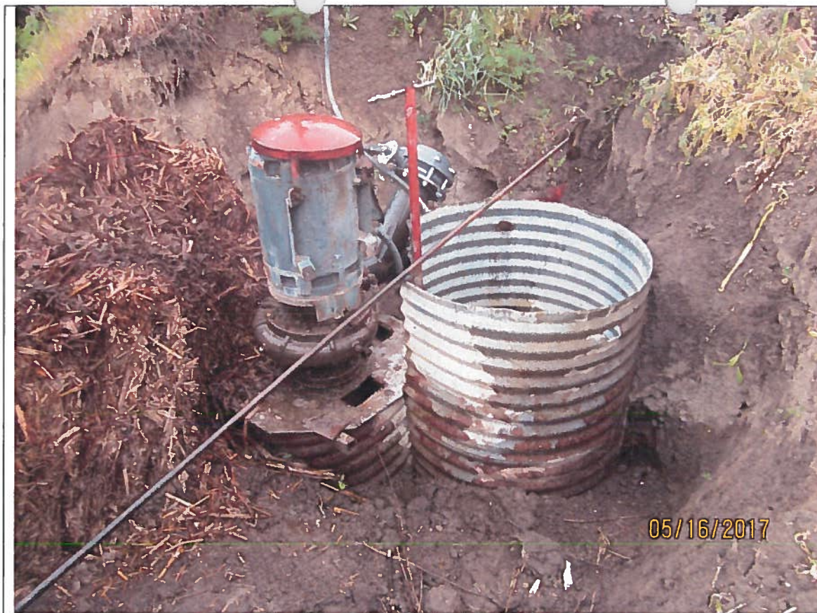
Looking at the POD from the east side of the creek.
