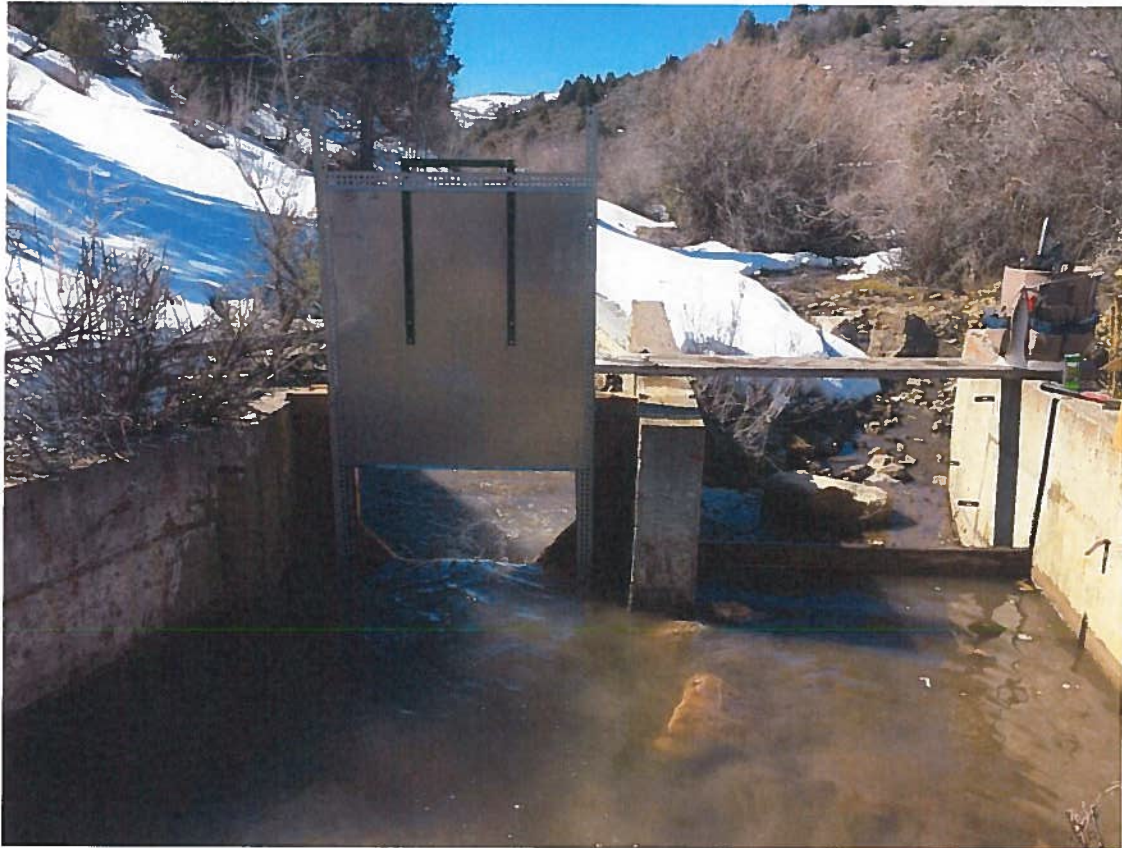
Figure 2 Example photo of slide gate.
