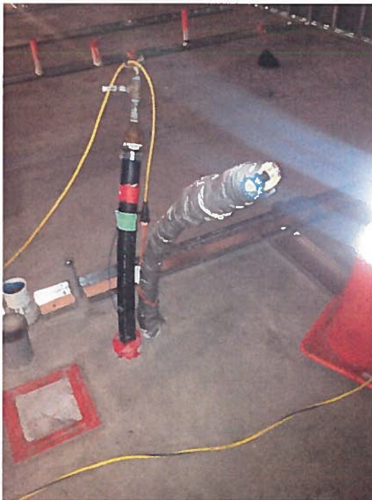
Figure 5 The control room where water is distributed to internal sprinklers to be used for fighting a fire.
