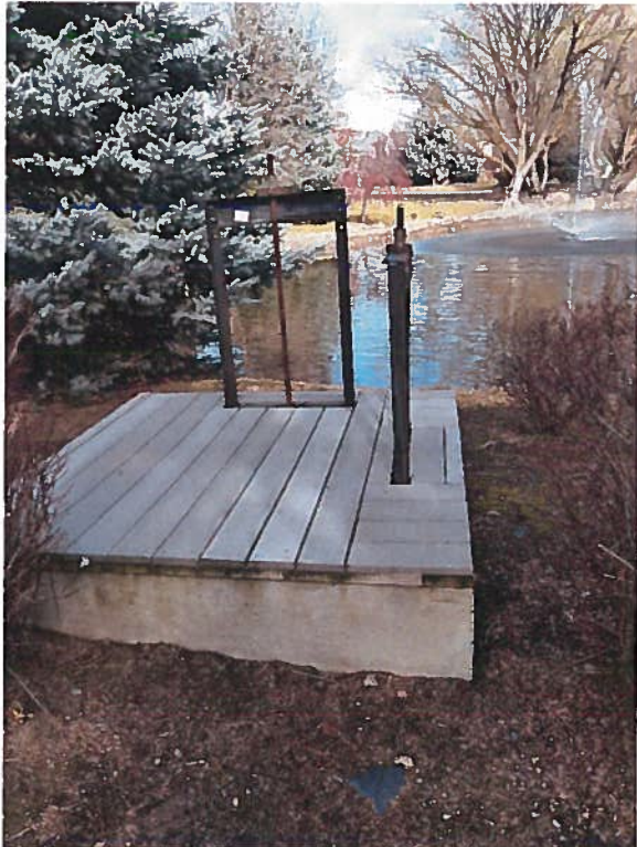
Figure 22 The headgate from the irrigation canal at the south edge of pond 1. Irrigation water is diverted into the system during the irrigation season. At that point, no groundwater is used in the system.
