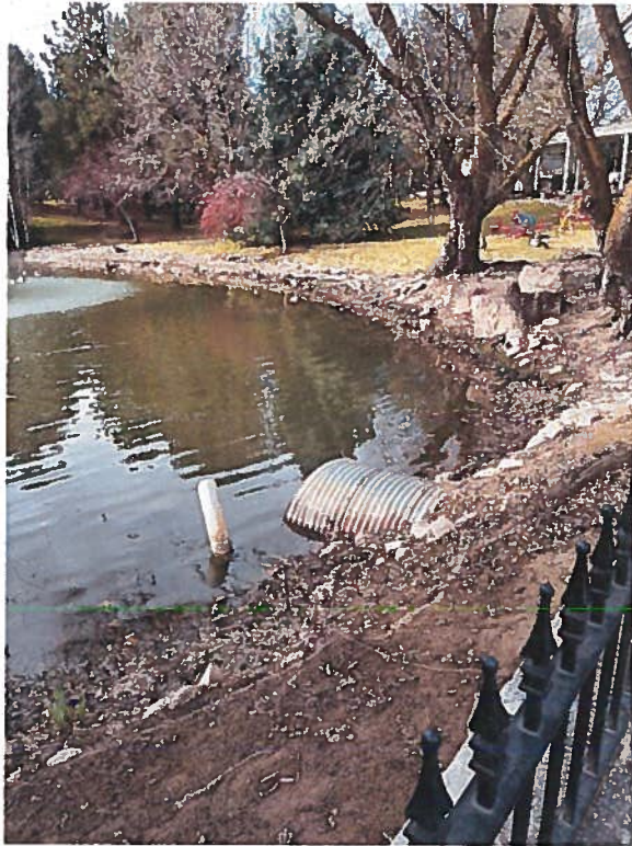
Figure 21 Pond 1, this pond is connected to pond 2 by a culvert which runs under the road. Irrigation water enters both this pond, and pond 16 at their southern borders along Floating Feather Rd.
