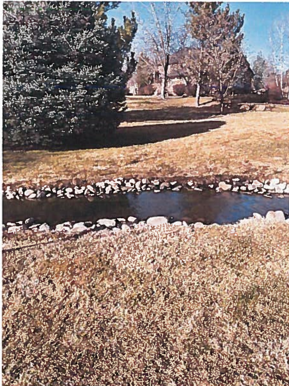
Figure 10 A typical length of channel between ponds. In general, the channel is around 2.5 ft wide with 4 to 8 inches of water.
