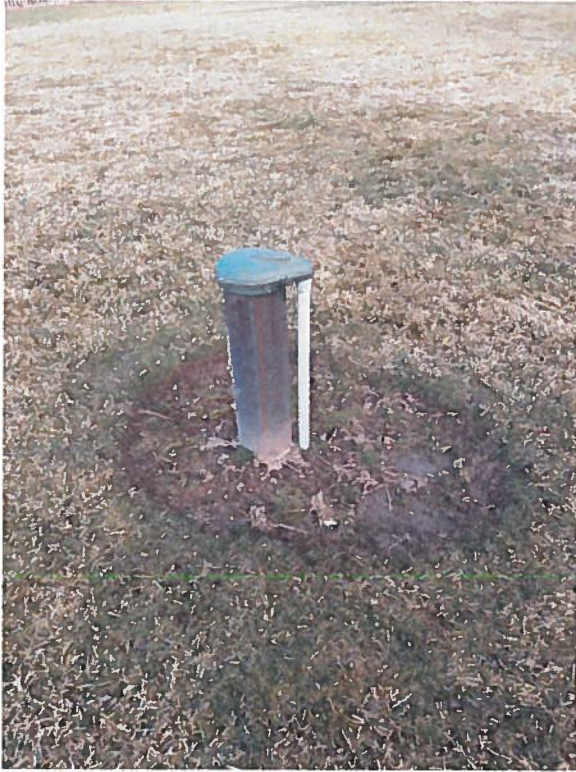
Figure 3 The 6-inch well at WPT 210.
