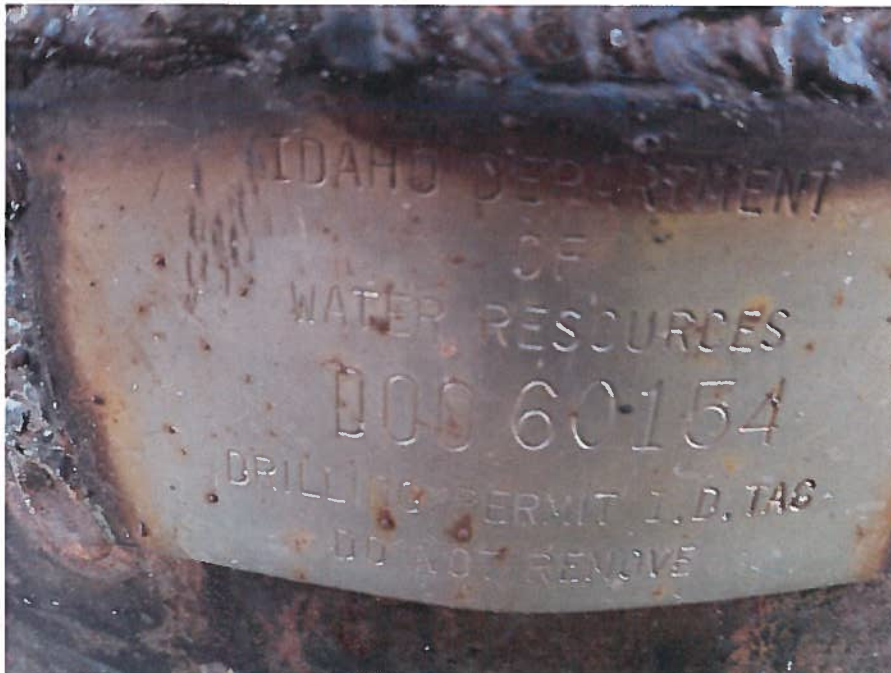
Figure 2 The metal tag for the fire protection well.
