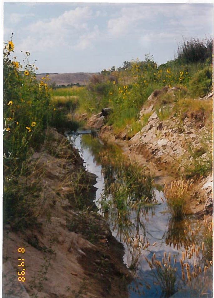
Photo 6 of 11: South down drain ditch
