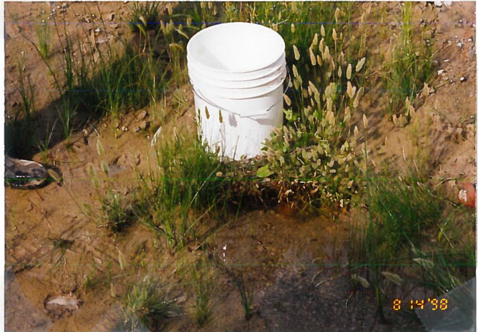
Photo 5 of 11: 6" culvert draining Quarter 5
