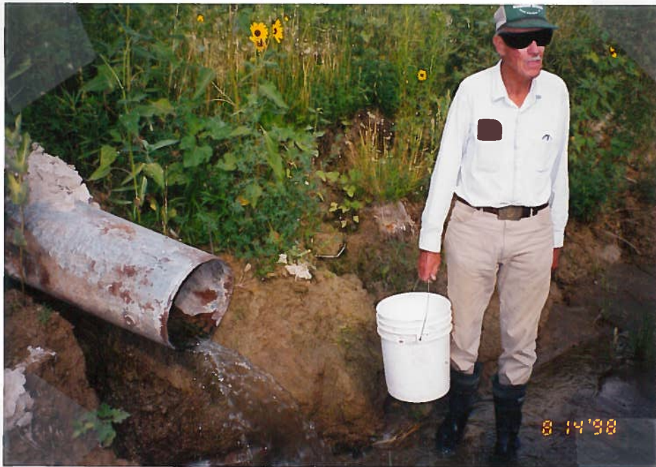
Photo 4 of 11: 12" culvert on N end of Res.
