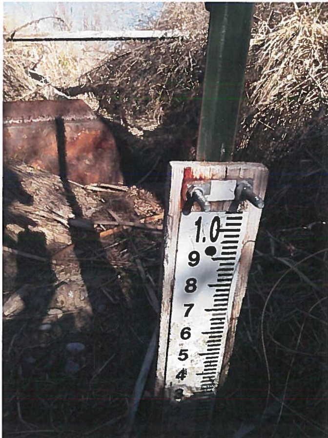
Figure 3 Water from the settling basin flows into the wetland through two separate cells. Before being discharged back into the drain.
