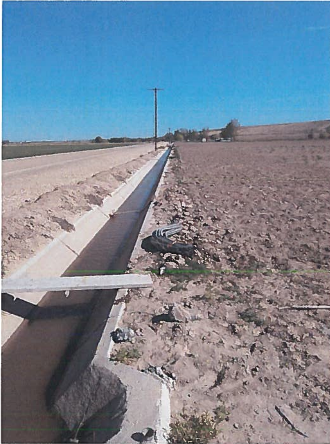
Figure 5 The owners use 1" siphon to pull water from the ditch and irrigate 59 acres.
