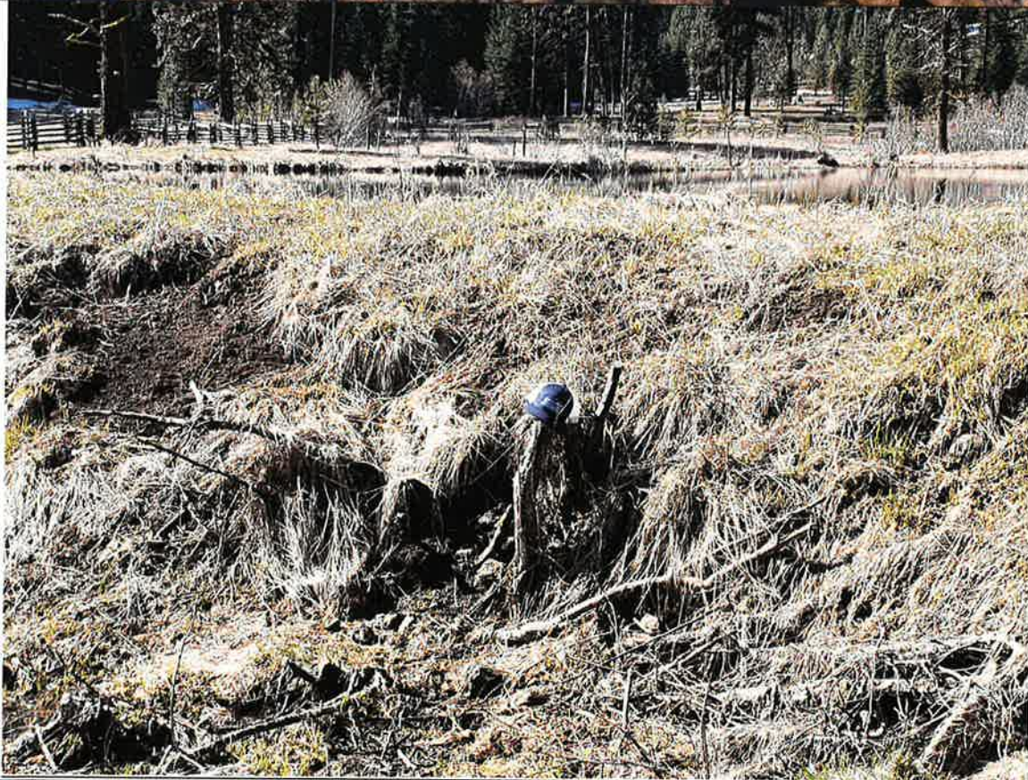
North side of the pond showing the built up embankment that creates the pond.
