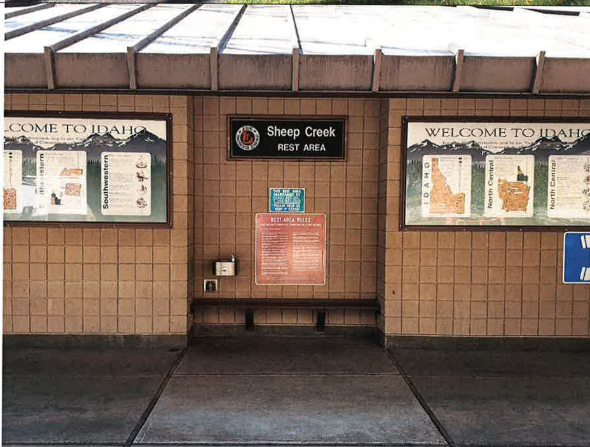
Entrance of the restroom area. Drinking fountain and hose bib shown in the picture.
