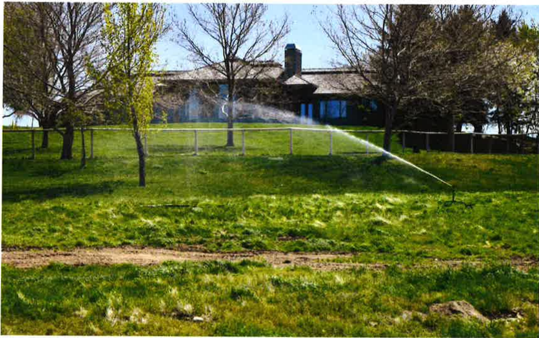
Movable big gun sprinkler on 2-inch hose between house and barn (April 2018 photo provided by Roger Cantlon)
