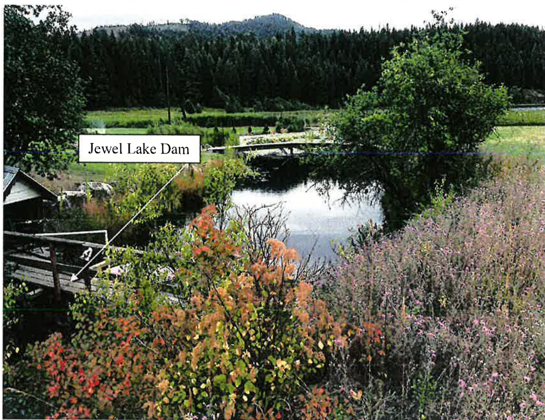
Photo 3 – Dam location (photo taken facing south)
