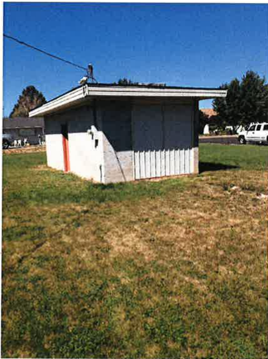
Figure 4 The pump house which contains the 2 storage tanks and the now-unused original well.
