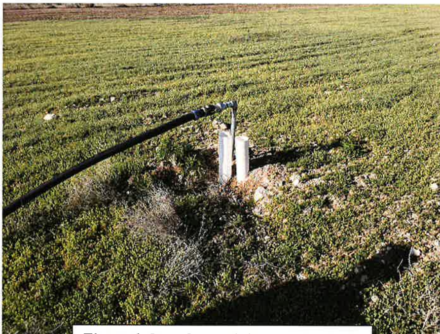
Figure 6 One of several risers used to hook up to K-Line.
