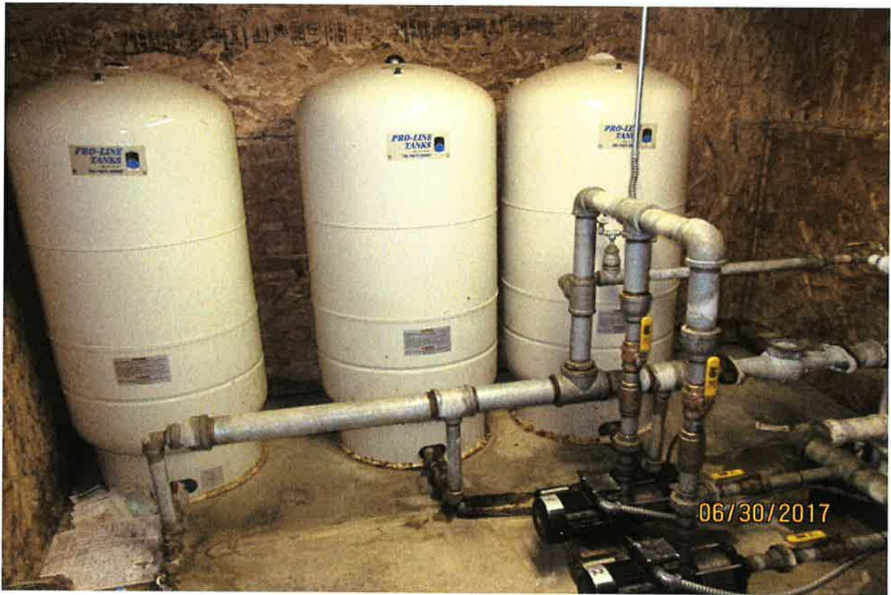
Water from the reservoir was then put into pressure tanks with two booster pumps for high demand.
