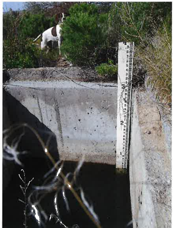
Water level behind V-notch weir after headgate diversion from Bruneau Buckaroo Ditch High water mark is shown at 0.93 feet
