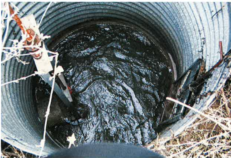
View inside box. Overflow slide gate on right. Diversion to pipeline on left.
