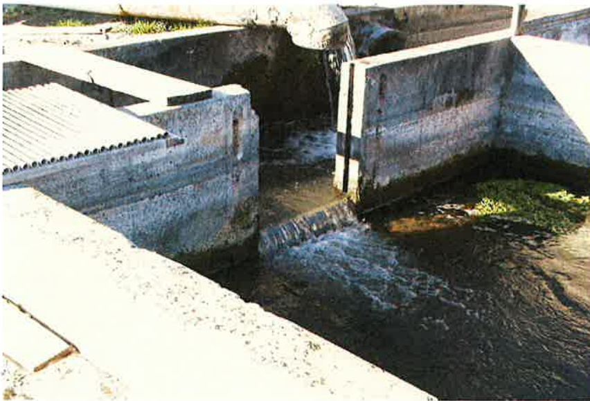
3' weir in head of raceway. Note concrete pipeline from Perrine Coulee in background is also off
