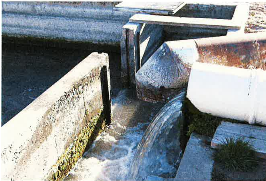
Flow from Porcupine Spring. Note pipeline from Alpheus Creek is off. Water measured through slot at head of raceway in background.
