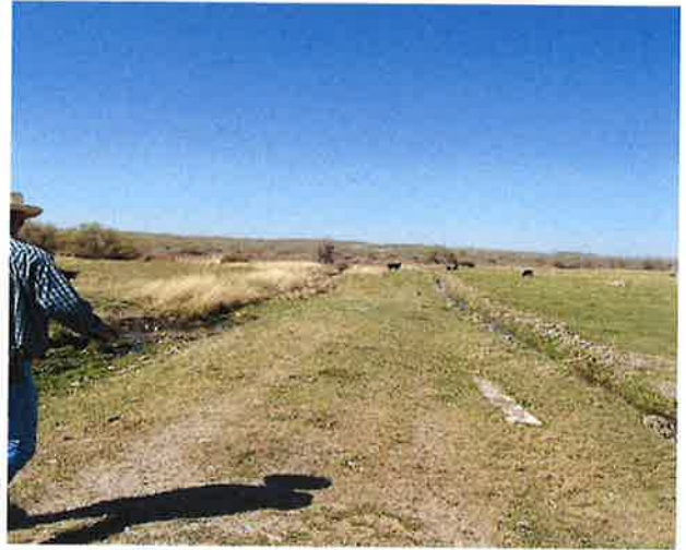
The ditch on the right is split from the main wasteway on the left and used to irrigate the field on the right
