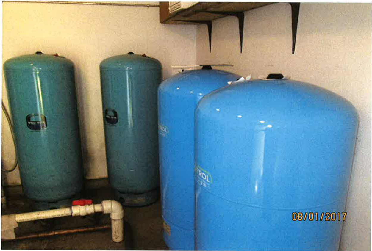
Pump house. Measurement was impossible due to storage tank and pressure tanks.
