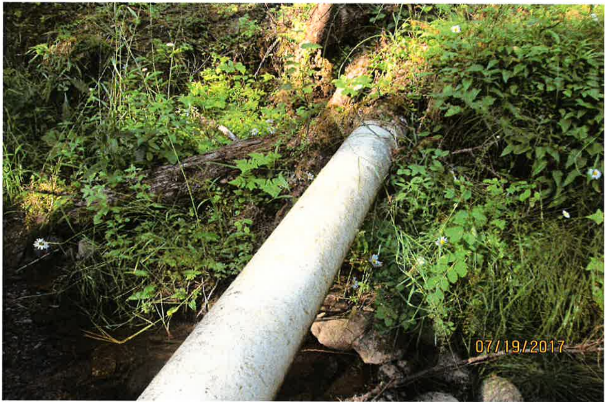
Proper measurement site half way down hill from POD.
