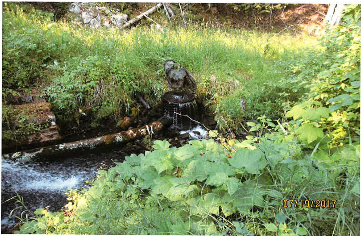
Just below dam, 8 inch pipe going to POU.
