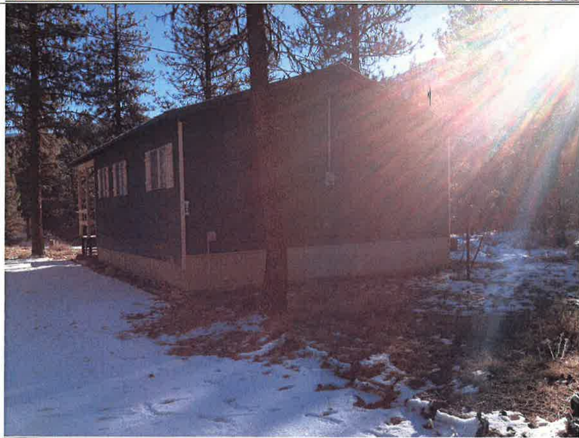
North side of the house looking south
