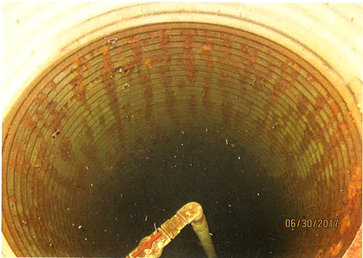
View inside culvert with 1 inch line.
