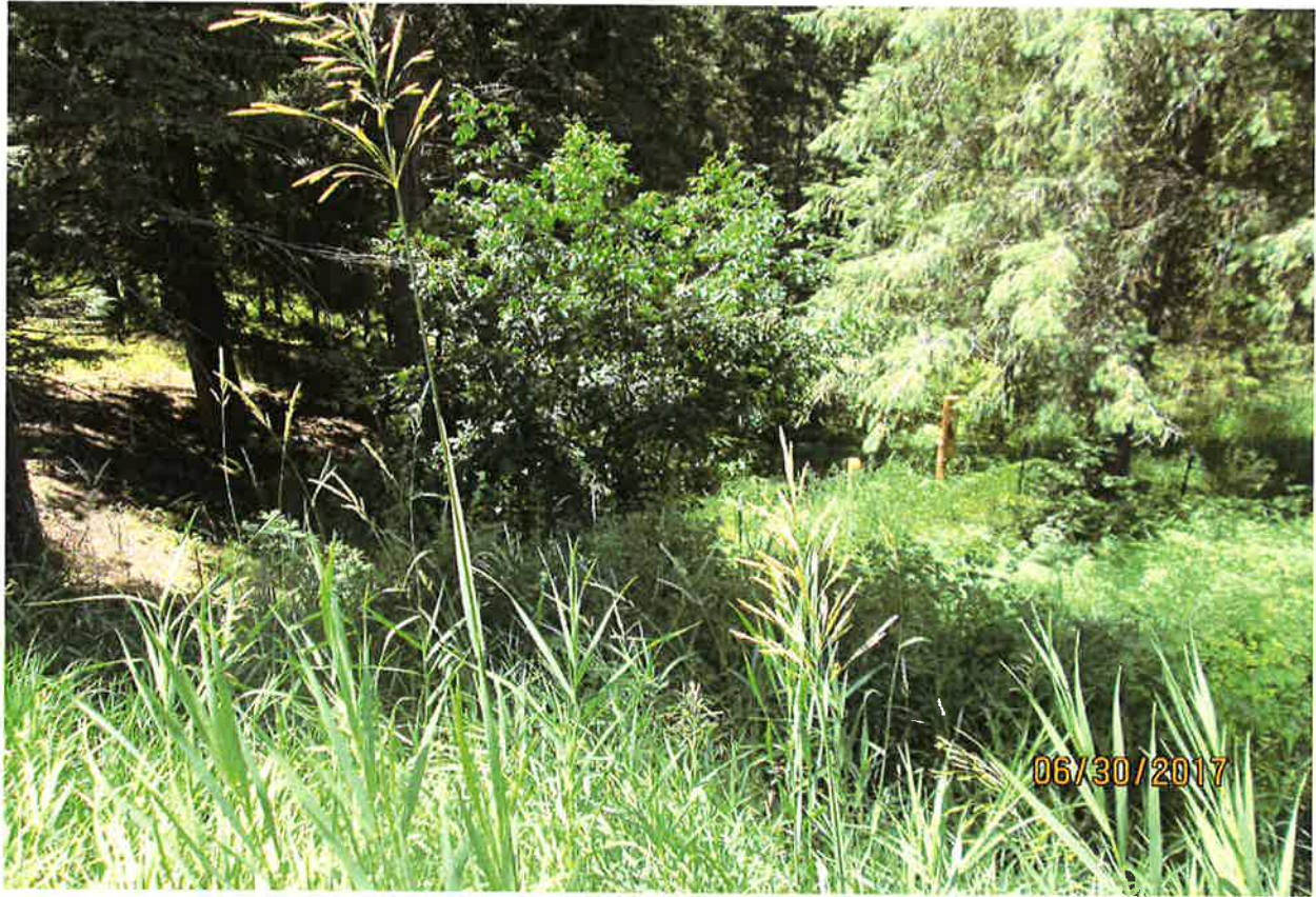
Creek looking downhill from dam and overflow pipe.
