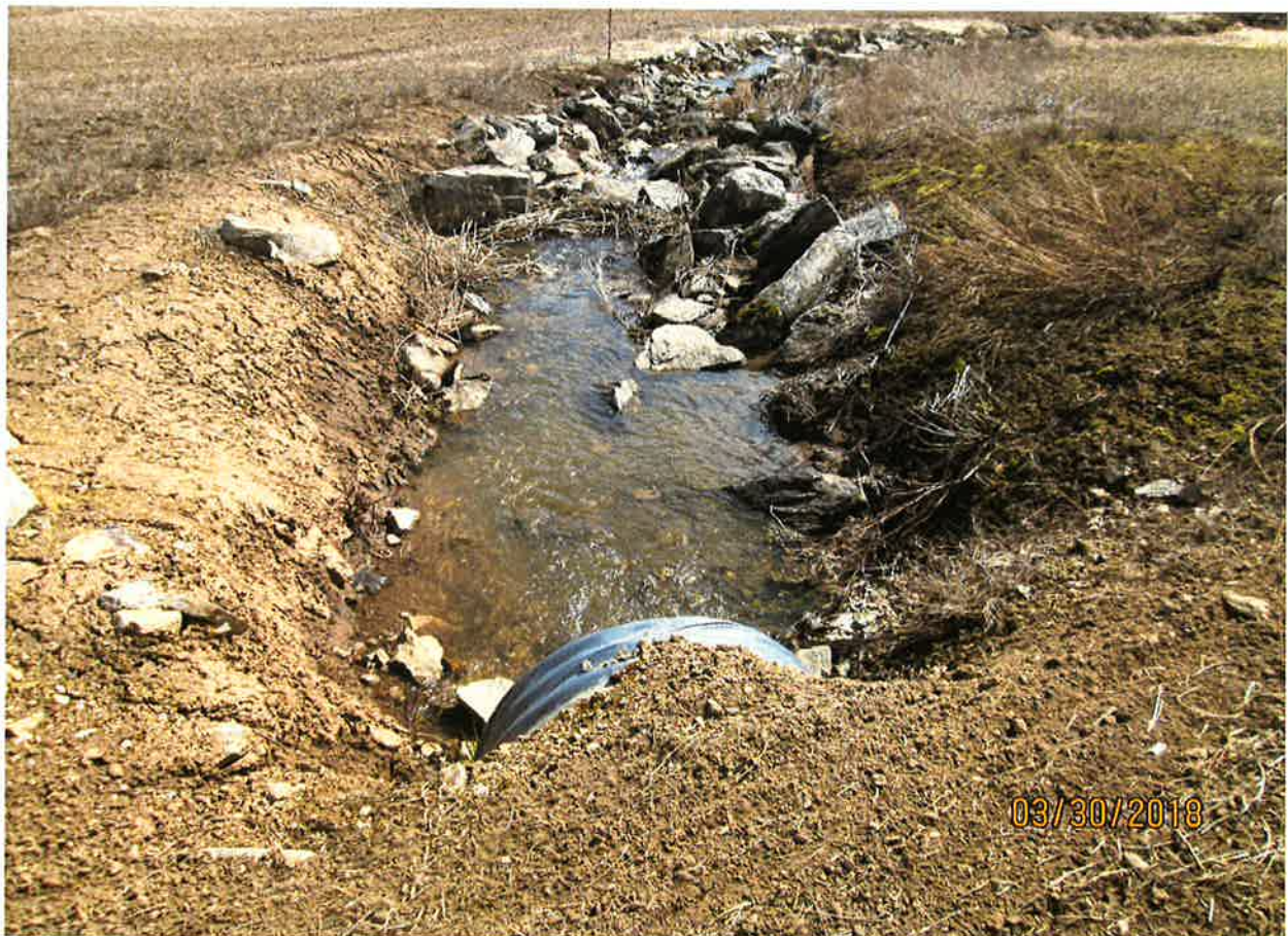
View downstream with end of culvert.
