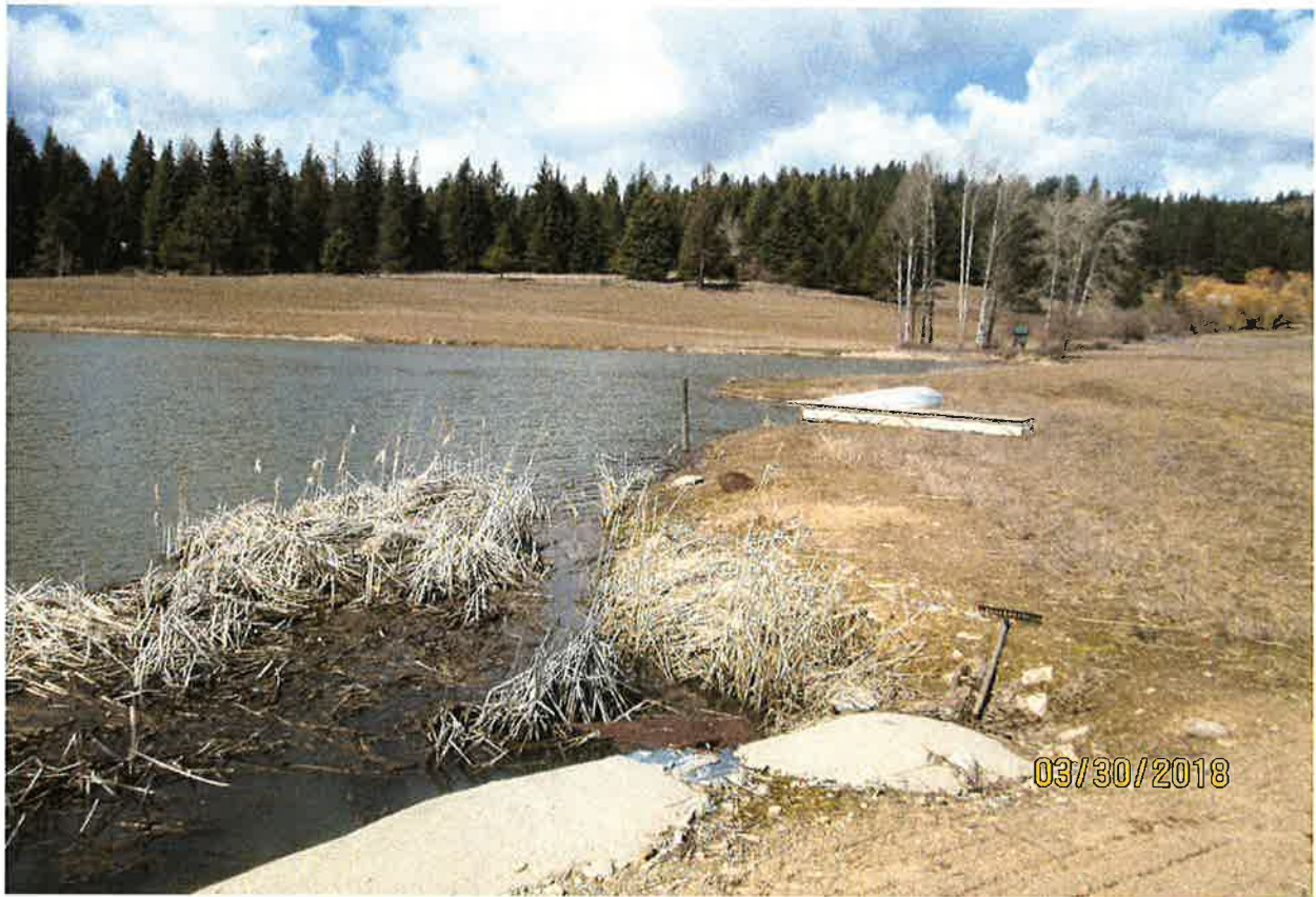
View of pond from dam.
