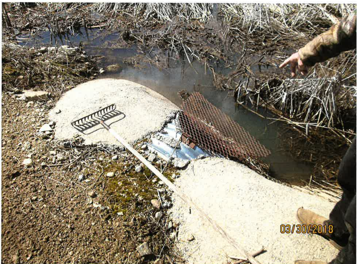
Outflow culvert at dam.
