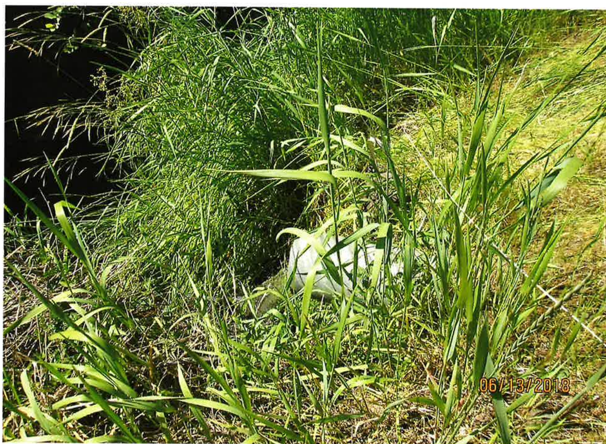
Outflow culvert flow back into stream.
