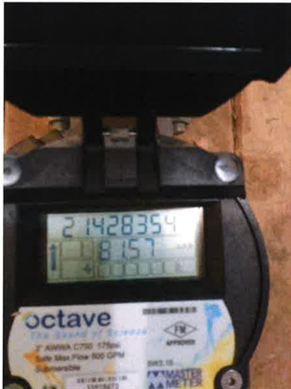
Figure 2 The Aurora in-line flow meter. Shown at 82 gpm while both K-Lines are running
