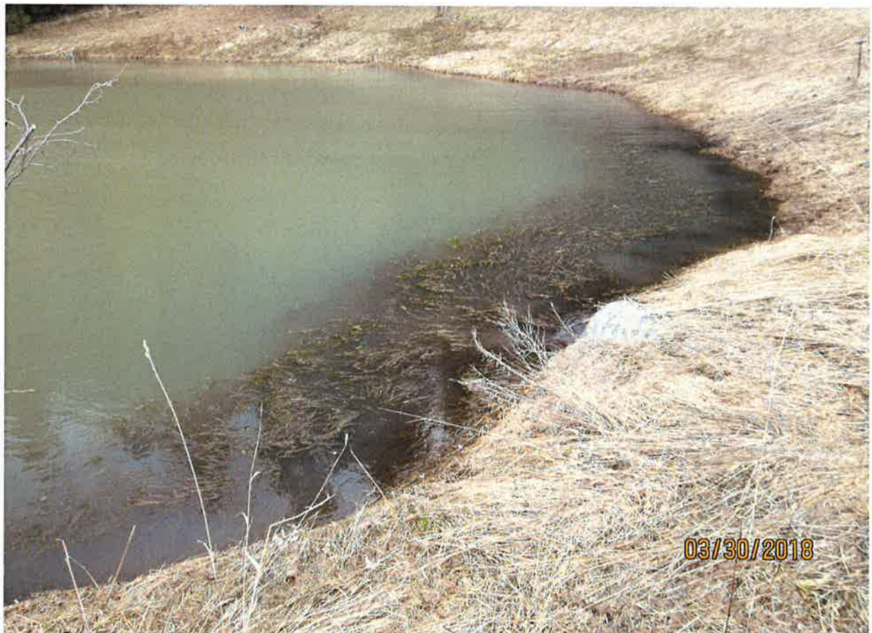
Looking at overflow culvert.
