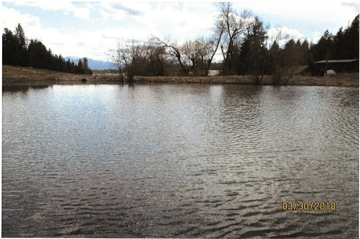
Pond taken from upstream edge looking at culvert and dam.
