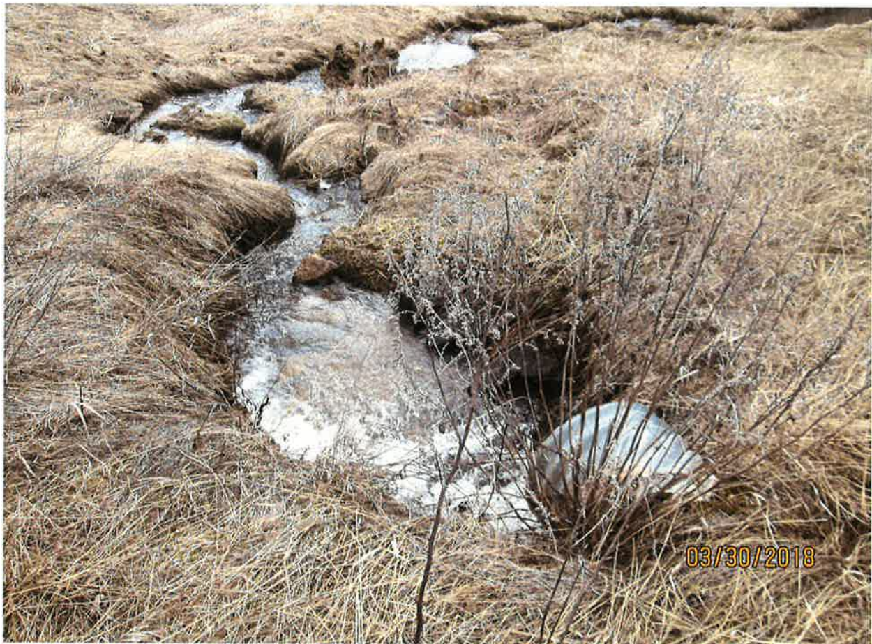
Outflow from culvert looking downstream.
