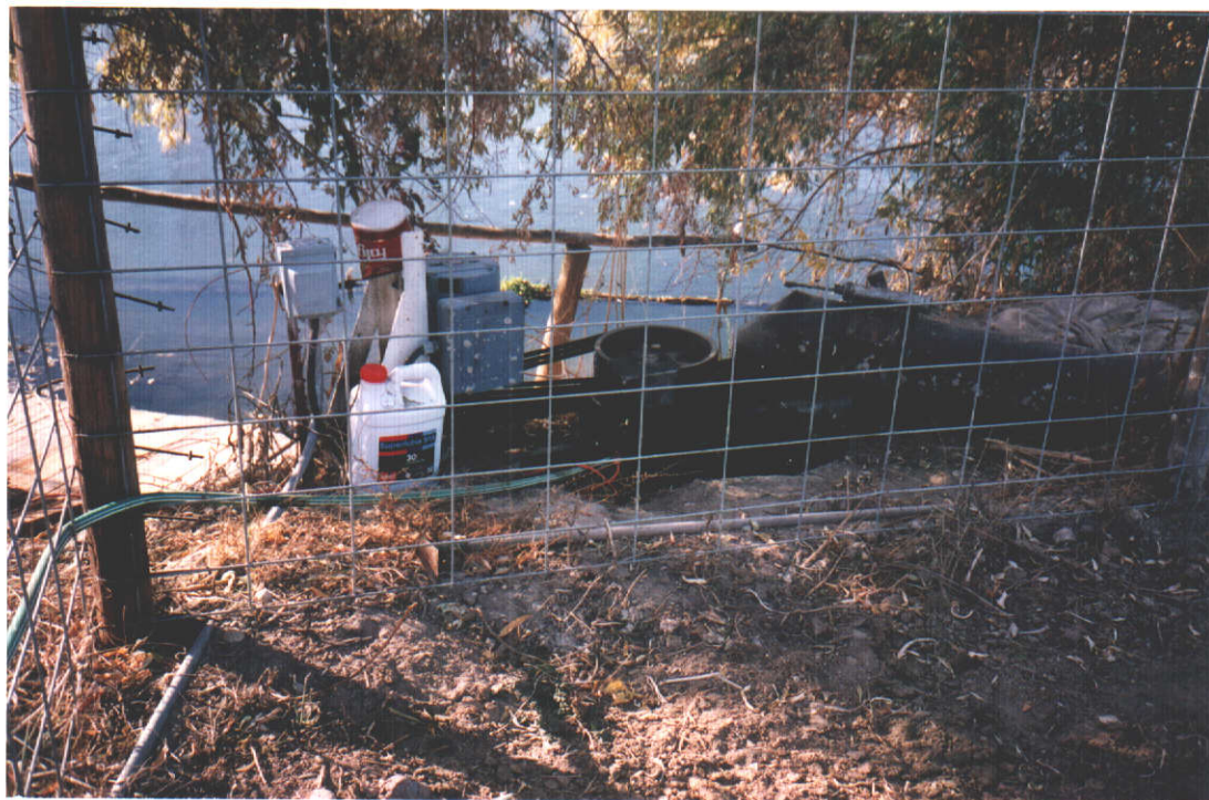
Schroeder's pump on river.
